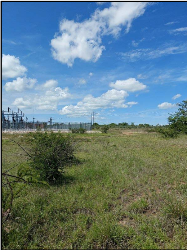
Figure 7.3. Image showing the existing infrastructure in the surrounding area.
