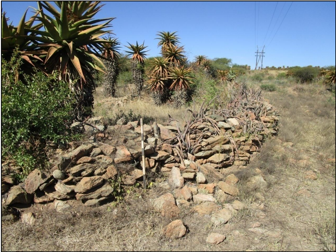
Figure 8. View of stone walling at feature 7.
