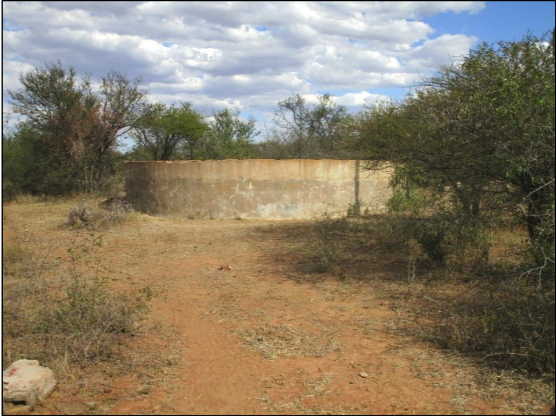
Figure 12. View of reservoir at feature 15.
