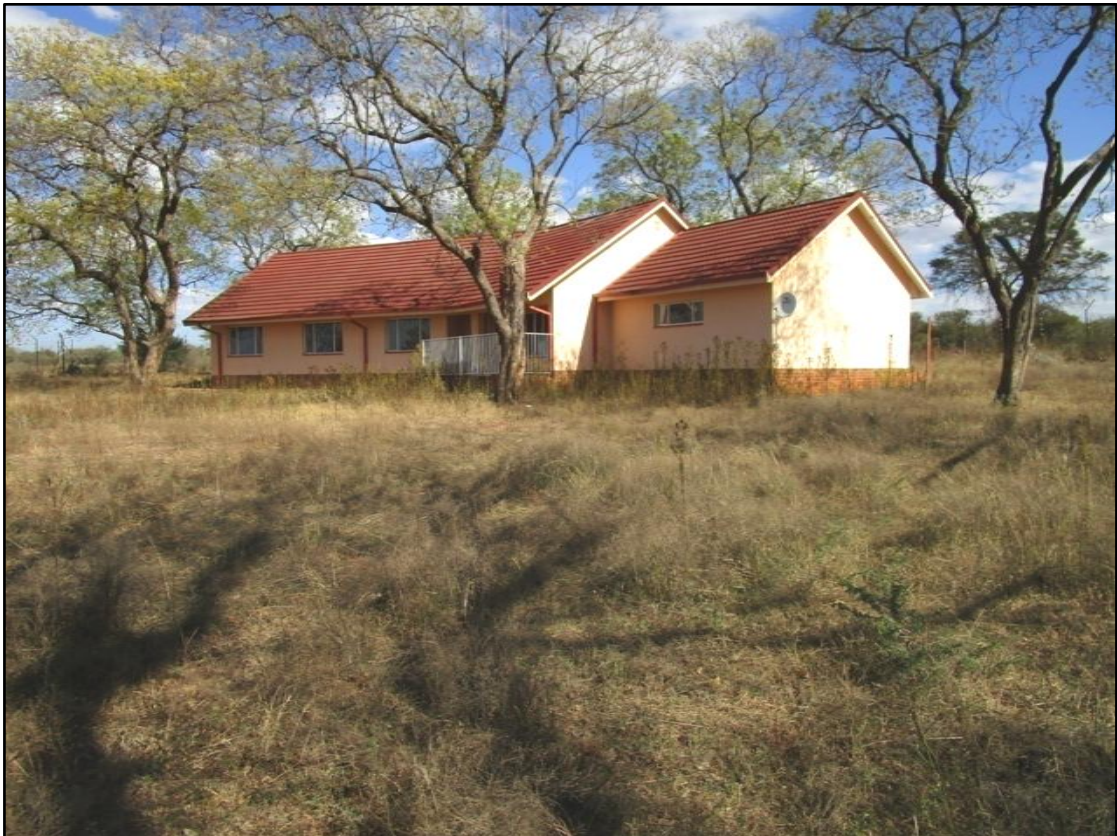
Figure 11. View of house at feature 14.
