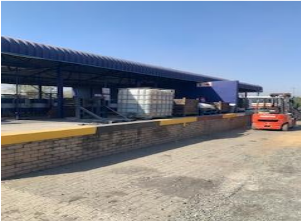
Figure 8: One of the recent buildings on site.
