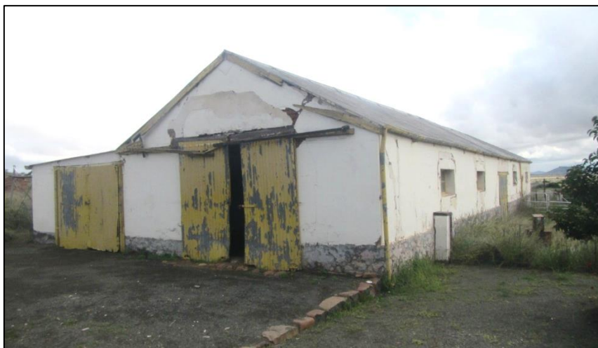
Figure 52: Outbuilding in the Basberg farm complex at waypoint 1023.
