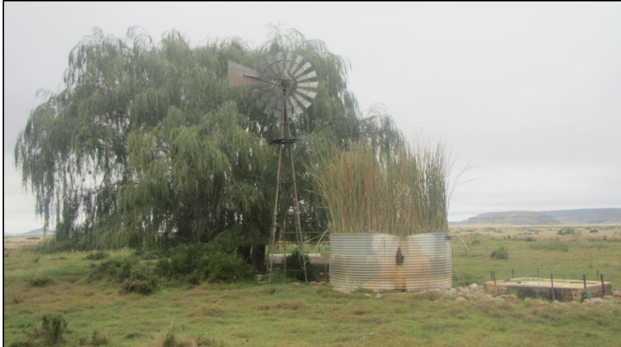
Figure 63: Waterpoint at waypoint 1014.
