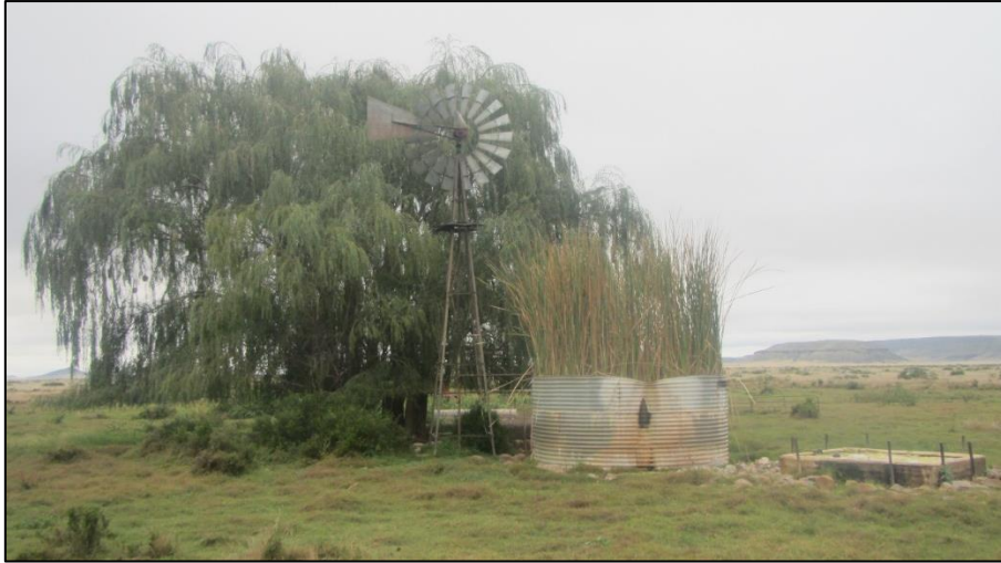
Figure 63: Waterpoint at waypoint 1014.
