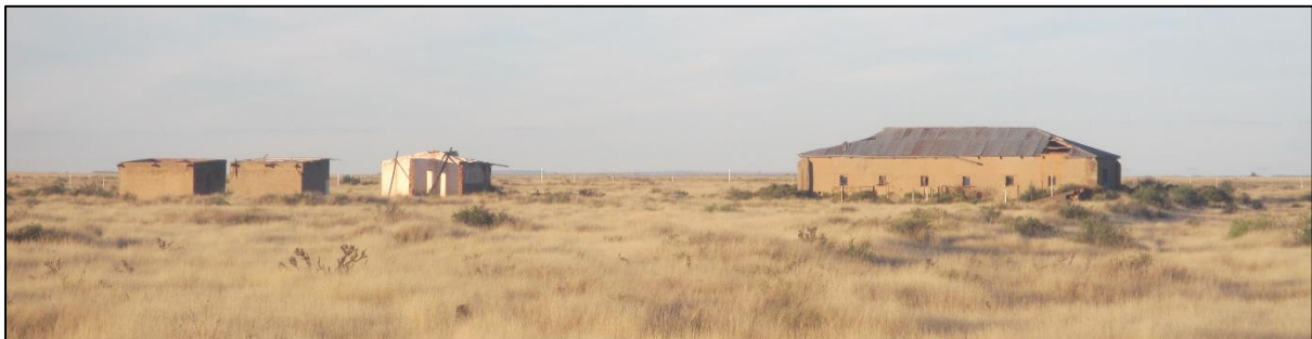
Figure 55: Structures/ruins at waypoint 983.
