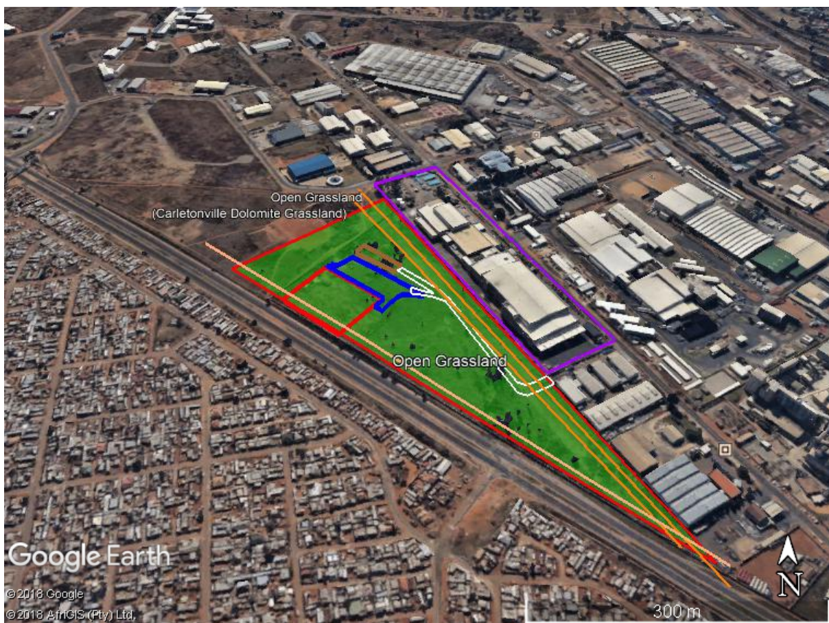
Figure 1: Google Earth map of the Adcock Ingram property on Clayville Ext 59. Map supplied by Texture Environmental Consultants.
