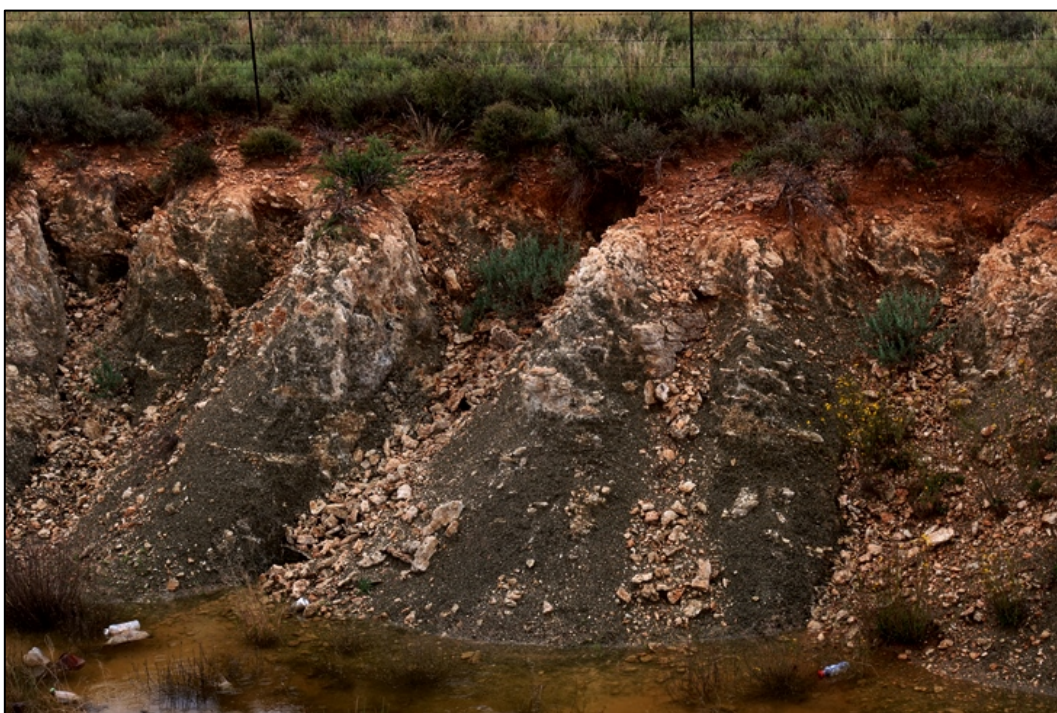
Figure 25: Good exposure of dark-grey, weathered, friable Tierberg Formation mudrocks showing extensive near-surface disruption and veining by Quaternary calcrete veins, seen here in an elongate roadside borrow pit on farm Grass Pan 1/40, c. 6.5 km west of and outside the Kudu renewable energy project area.
