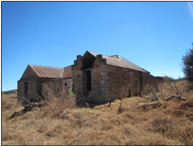
Figure 20 – Historic structure at ILM003
