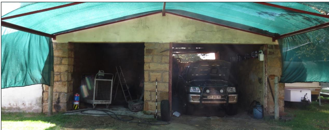
Figure 28 – General view of the structure.
