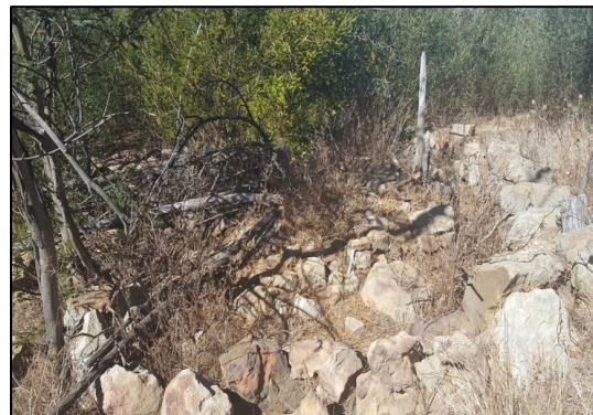
Figure 27 – Clear view of outer wall enclosing an inner pile of smaller packed stone.
