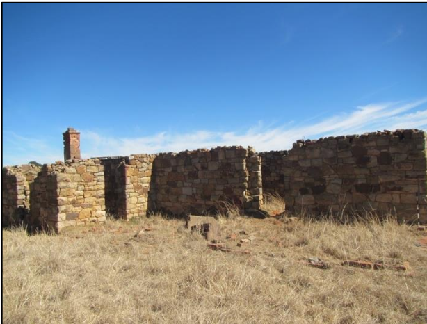
Figure 28 – General view of the main structure from behind.
