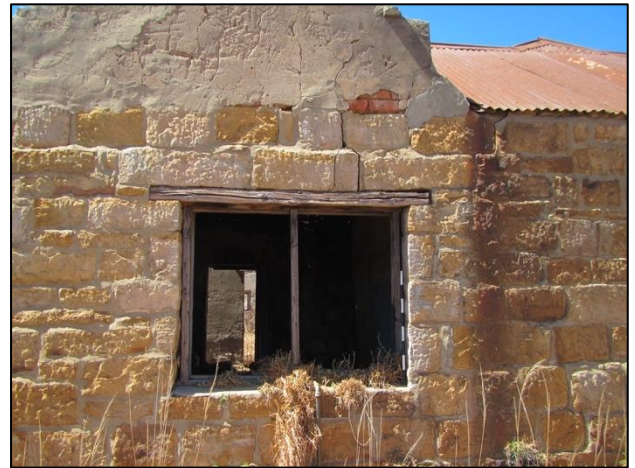
Figure 21 – Building style and alterations at ILM003
