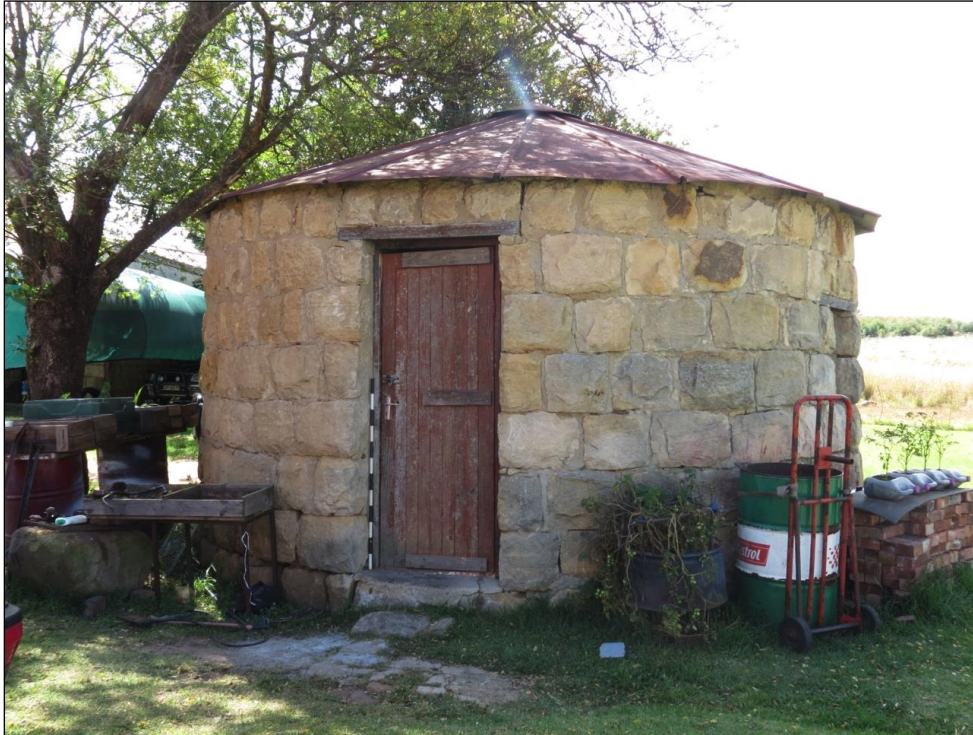
Figure 26 – General view of the rondavel structure. Note the lintel, door and doorframe all manufactured of wood.
