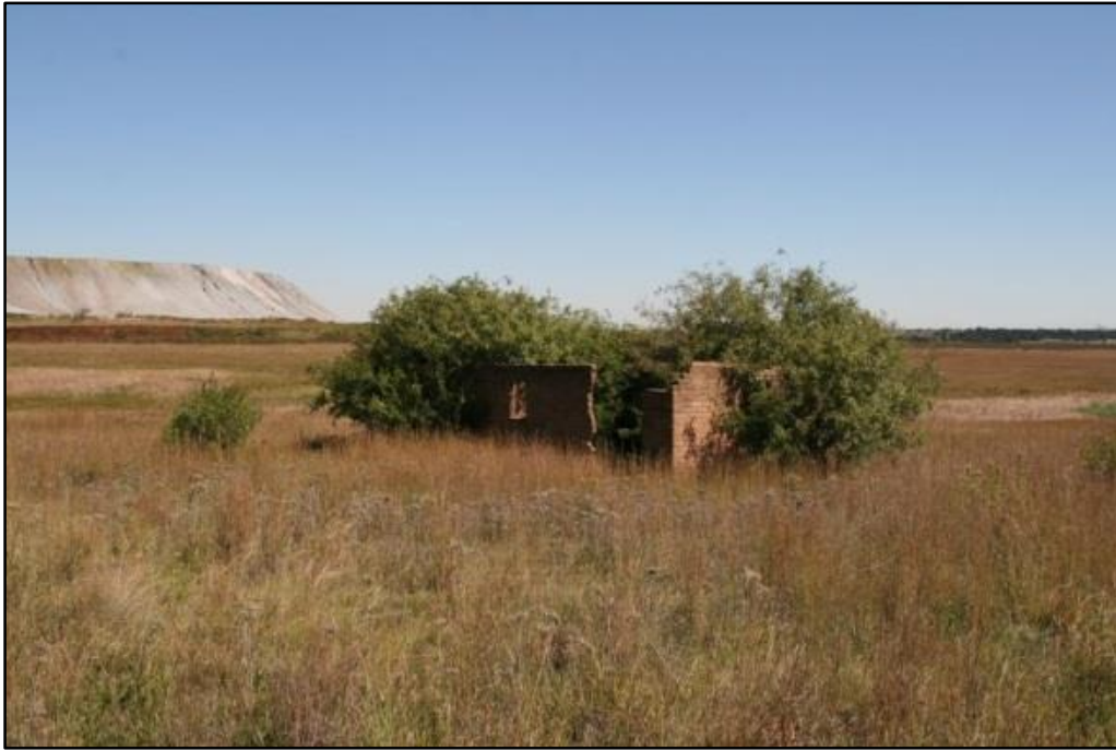
Figure 11 – Structure as viewed from the east towards the existing ash dump
