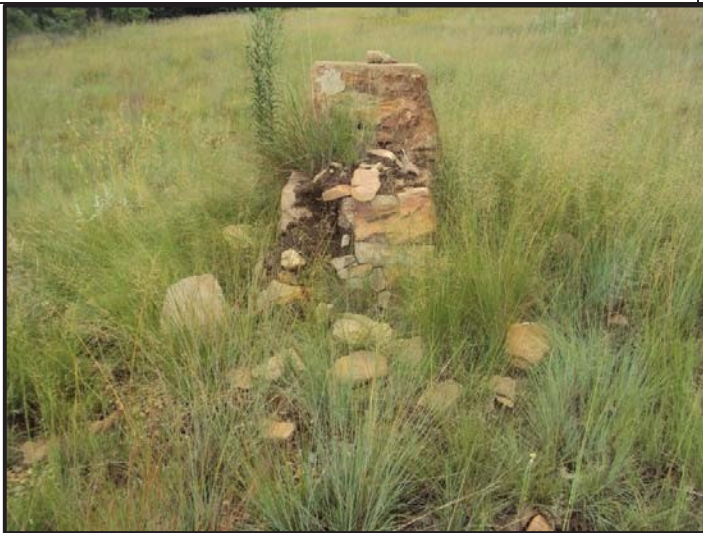
Figure 7. Demolished remains of structures (Photo S. Ingle)
