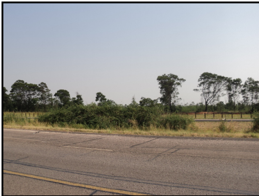
Figure 6: Site of N4 highway crossing.
