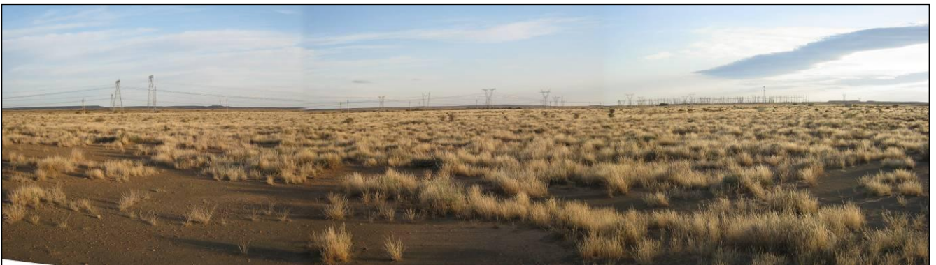
Figure 7: View southwest from the middle of Alternative 3. Note the power lines leading from east to west to the substation on the far right hand side of the photograph.
