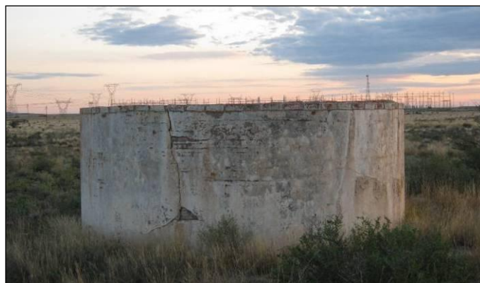
Figure 25: The small cement and brick dam on Alternative 3.
