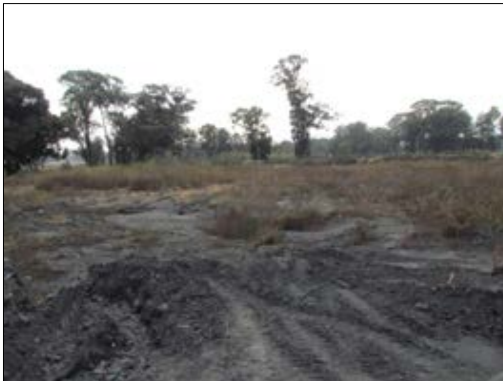
Figure 7-3: Eastern End of the Re-alignment Located next to Dump
