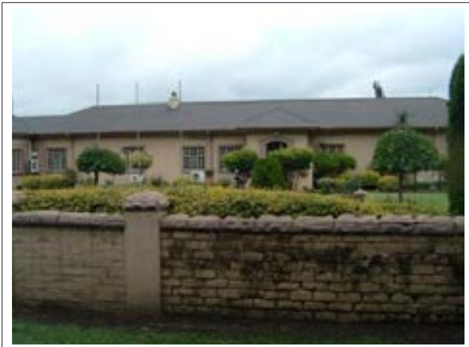
Figure 28- XSA administrative office complex possibly includes individual structures or a core which may qualify as historical significant (above).
