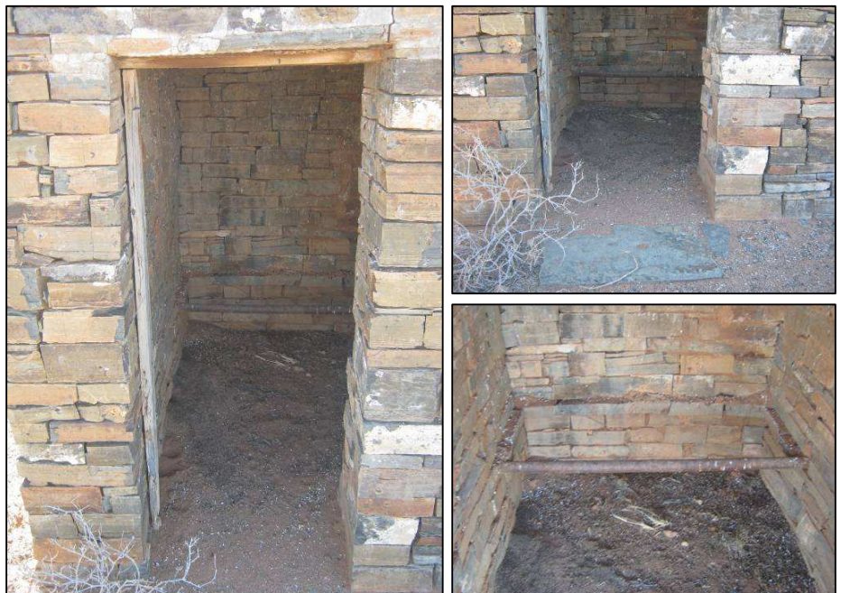
Figure 57: The doorway of the toilet house at KGP2011/019 (#040).
