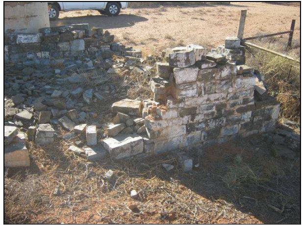
Figure 44: The same ruin as Figure 43 but viewed from the other side showing a white-washed wall.
