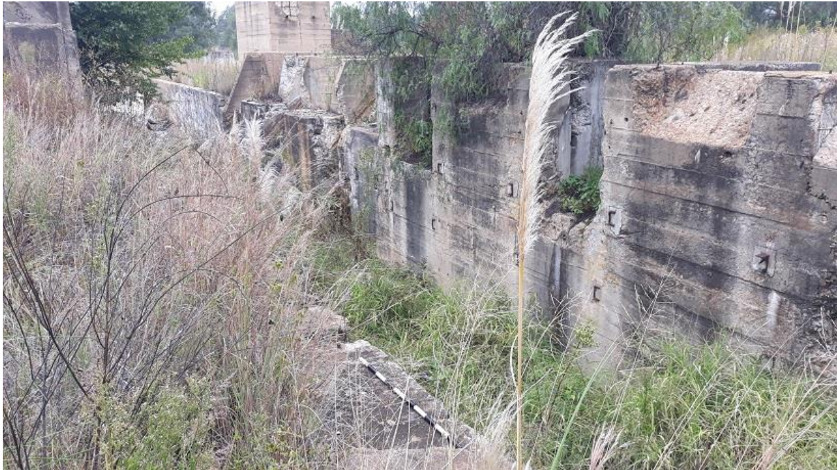
FIGURE 22: REMAINS OF CONCRETE CHANNELS AT SITE 3.
