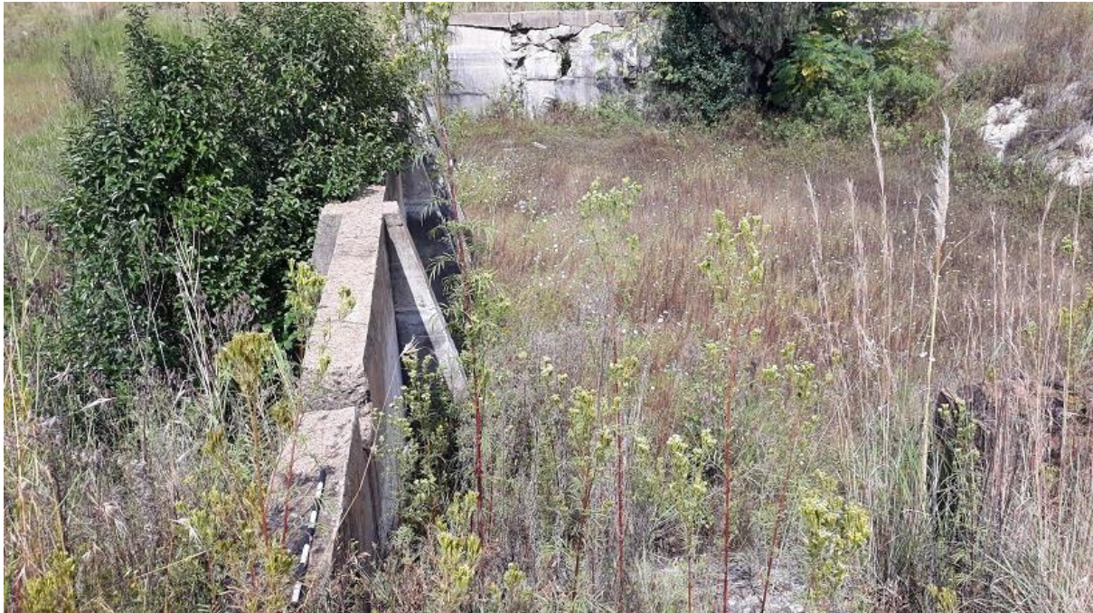
FIGURE 20: OLD DAM LOCATED AT SITE 2.
