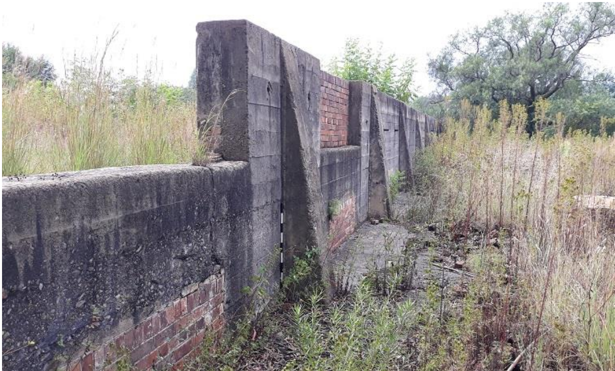
FIGURE 21: WALL YOUNGER THAN 60 YEARS AT SITE 2.
