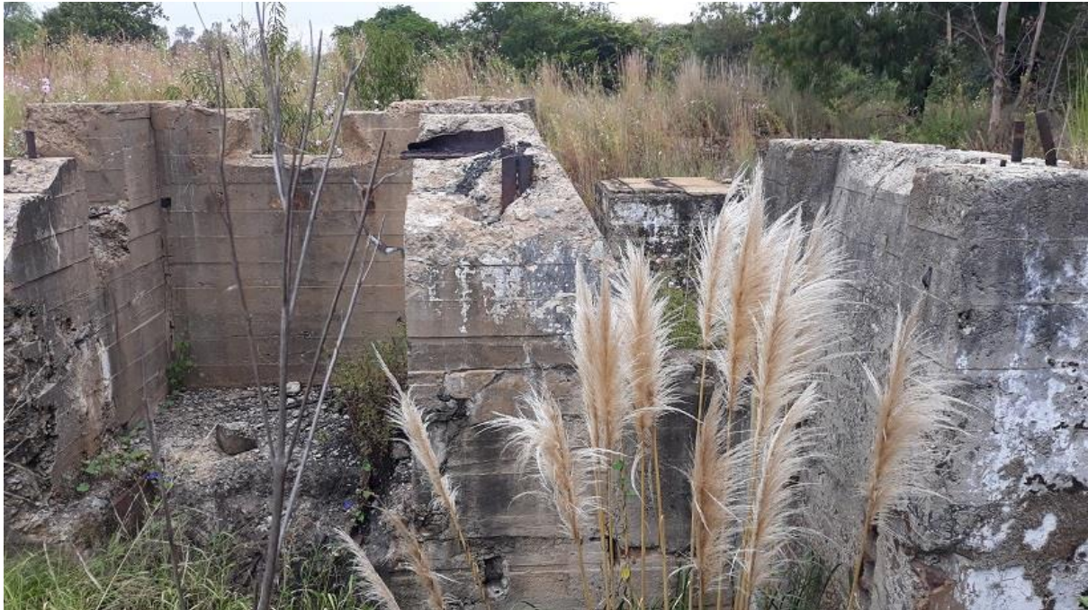
FIGURE 6: OLD MINING INFRASTRUCTURE AT THE TSF EXPANSION WEST.
