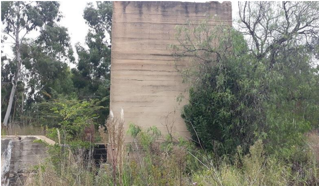
FIGURE 23: LARGE CONCRETE STRUCTURES LOCATED AT SITE 3.
