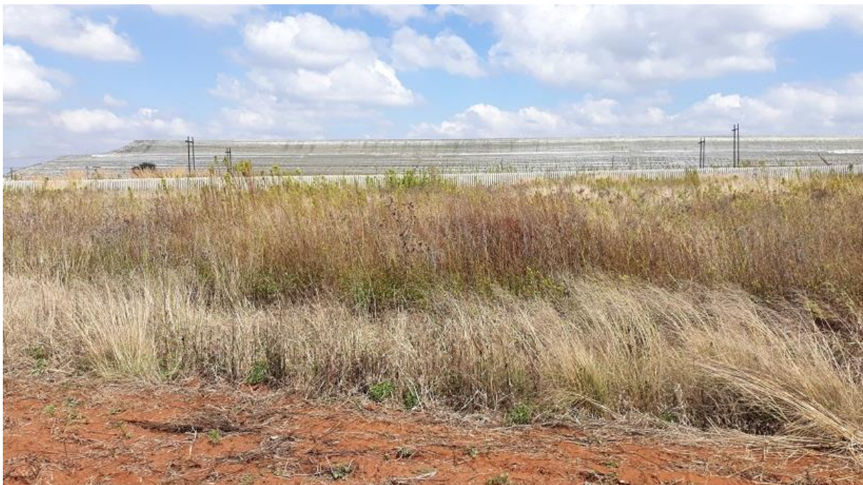
FIGURE 7: MINING INFRASTRUCTURE AT THE TSF EXPANSION NORTH.
