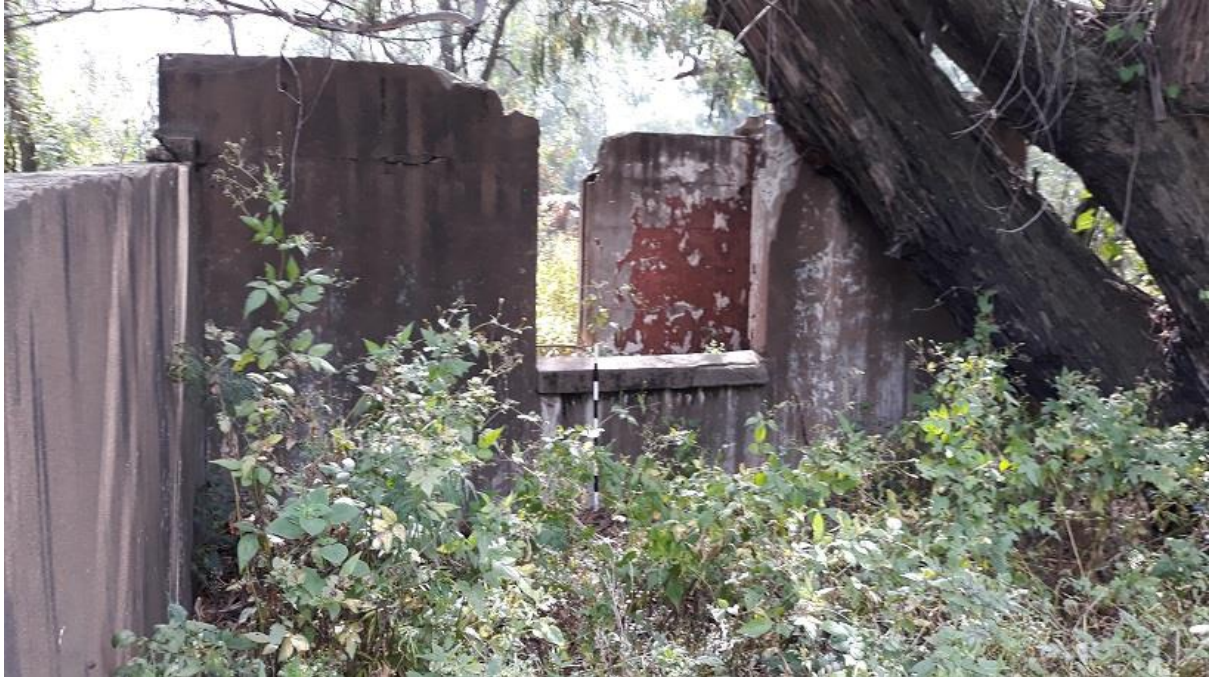
Figure 15: STRUCTURE OLDER THAN 60 YEARS OF AGE AT SITE 1.
