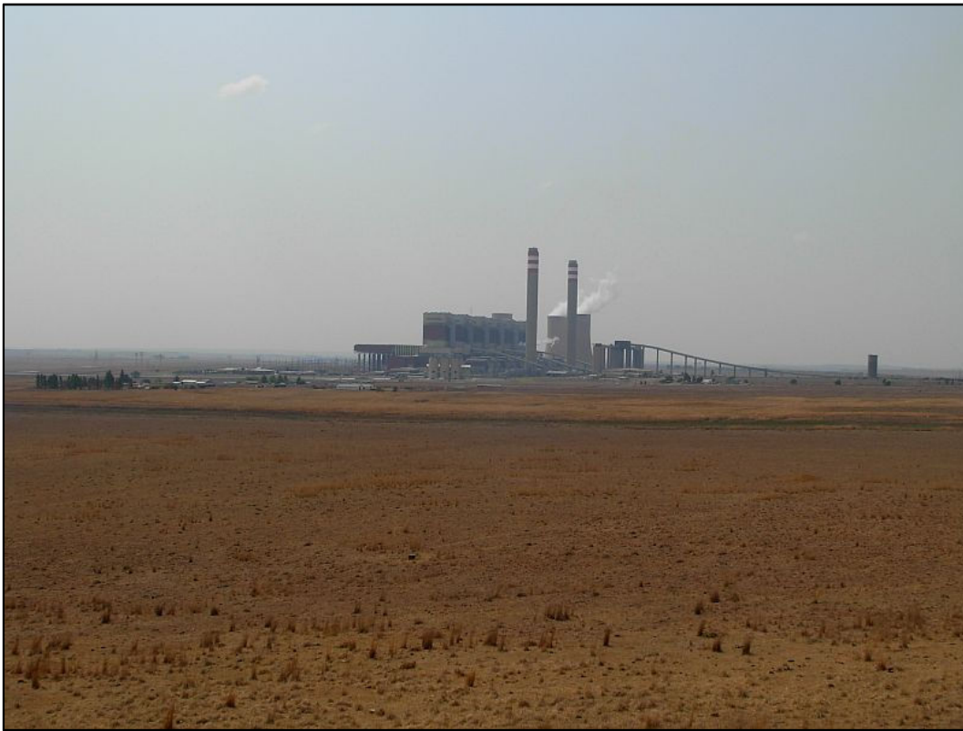
Figure 5 - Majuba Power Station in north western corner of study area
