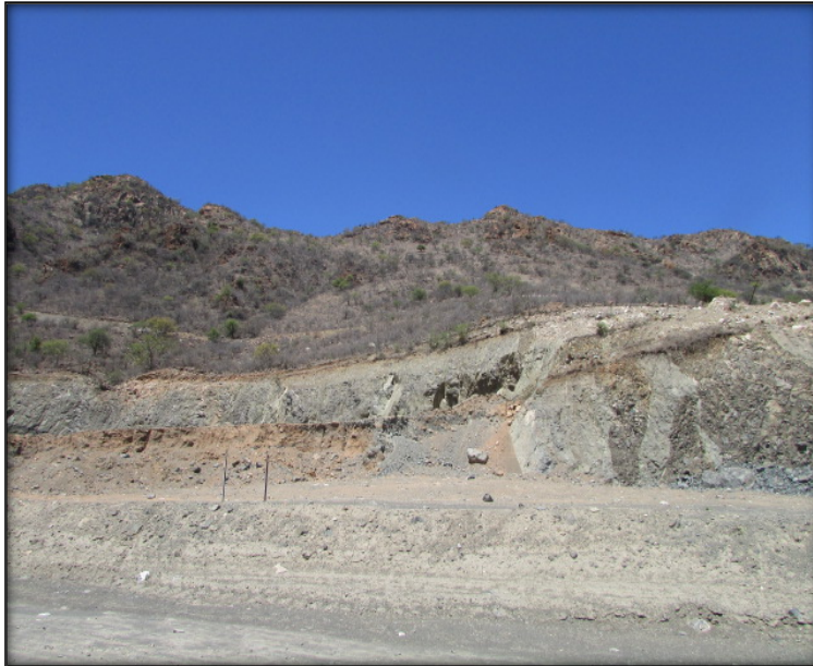
Fig.8: Further view of the existing mining's impact.
