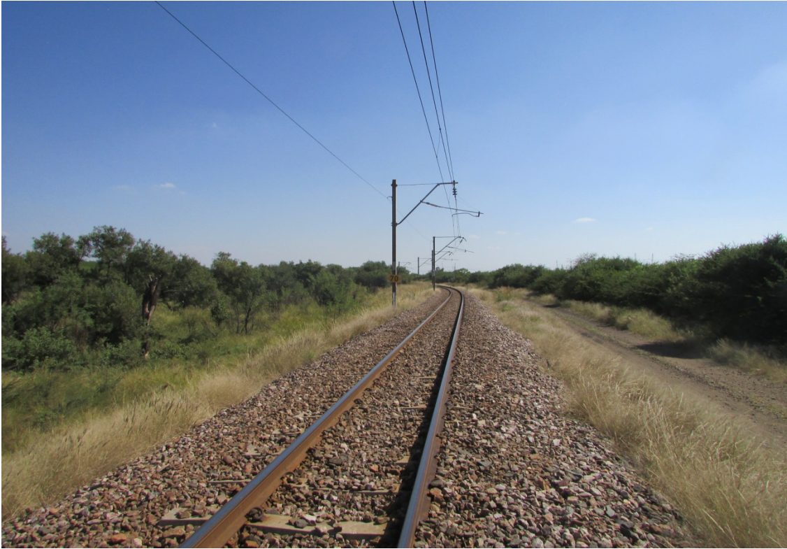
Figure 12: A view of a section of the railway line that cuts through part of the area.
