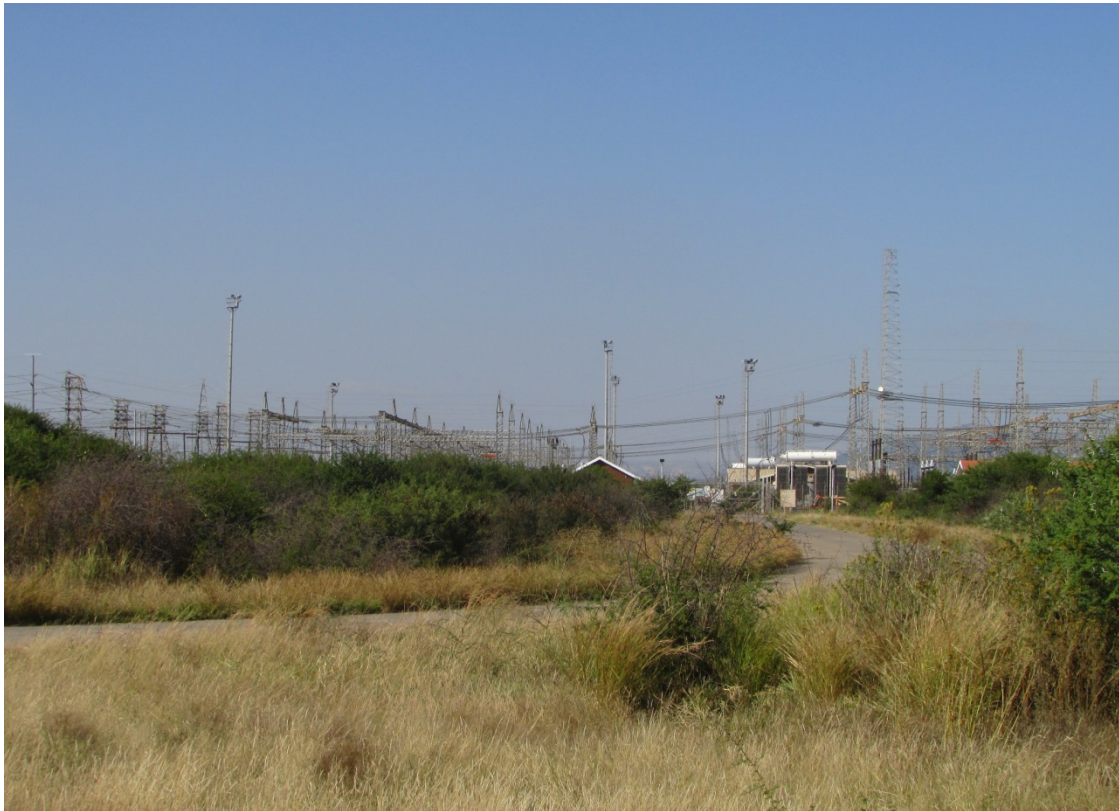
Figure 5: Picture of Eskom substation in the area.
