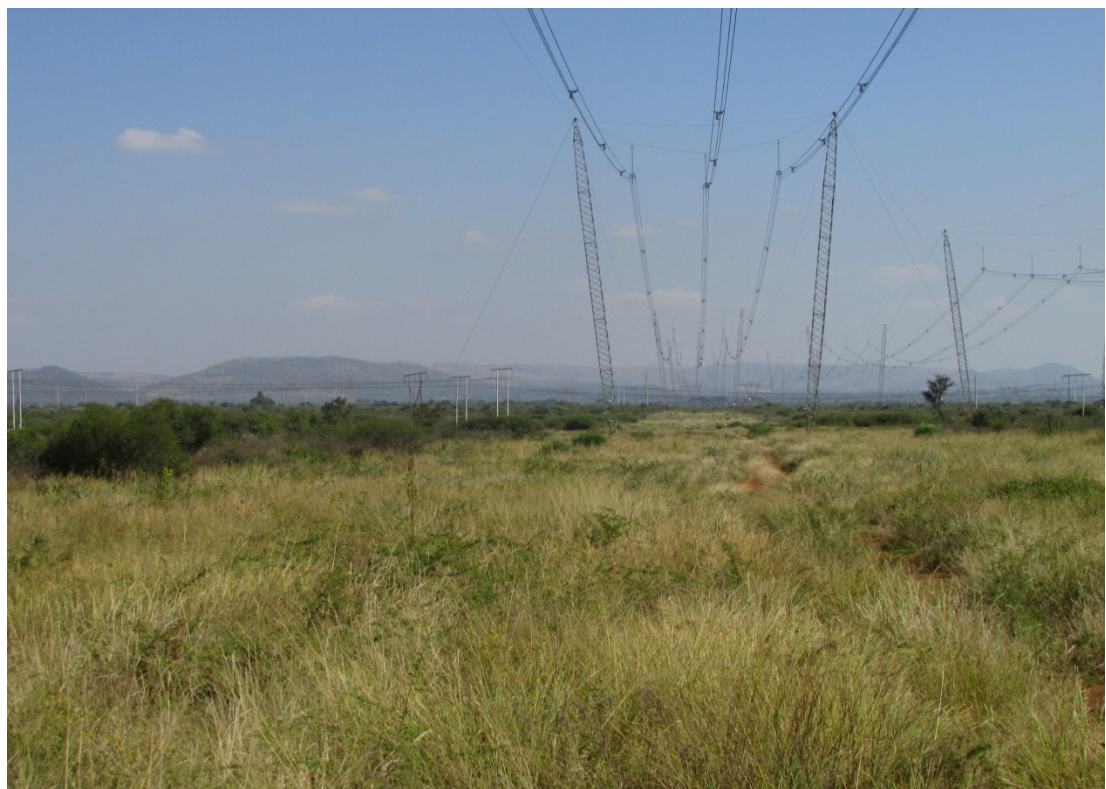
Figure 11: Another general view of the area with the impact of the Eskom Powerlines & Pylons evident.
