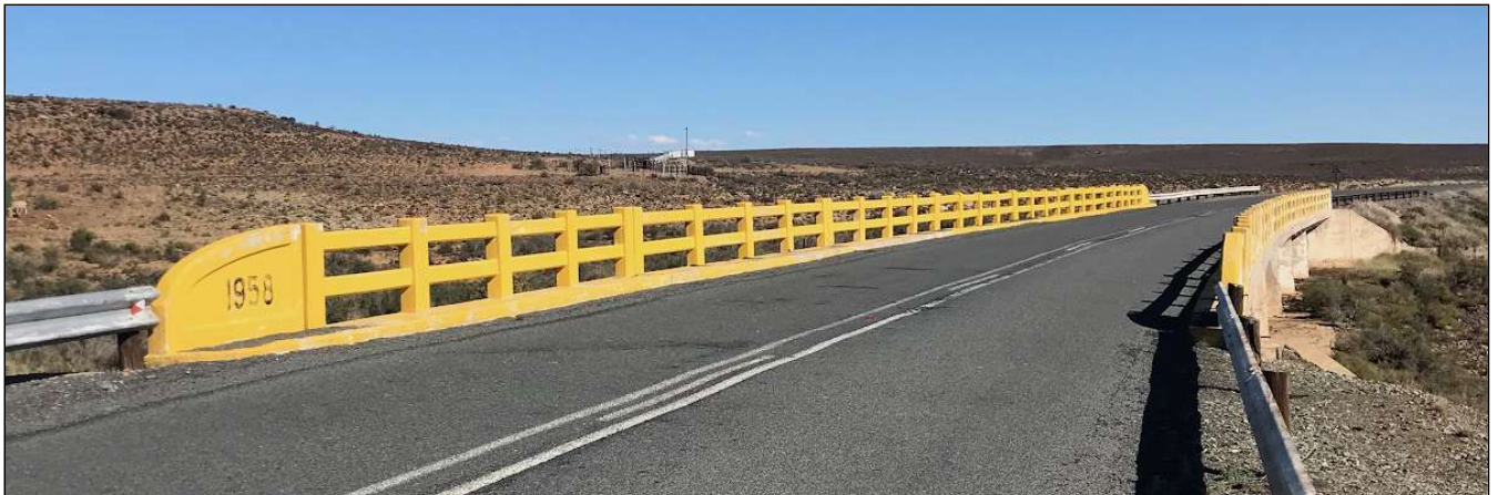
Figure 6.5 BTC07 - Bridge over the Soutpoot River (1958)
