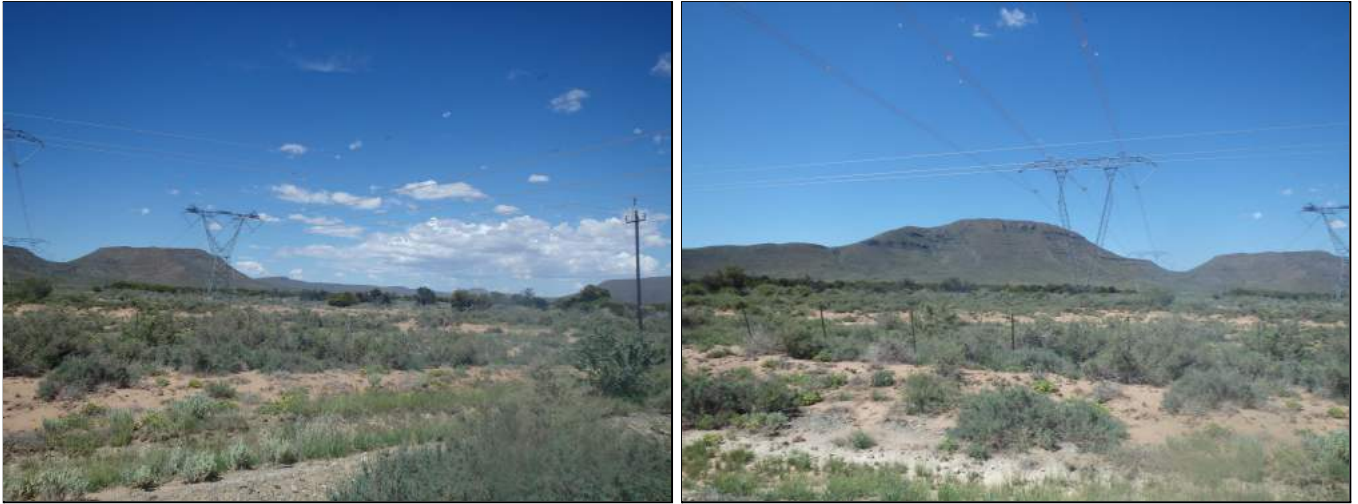
Figure 4.2: Existing grid infrastructure lying to the east of option E with views of koppies near Nelspoort.
