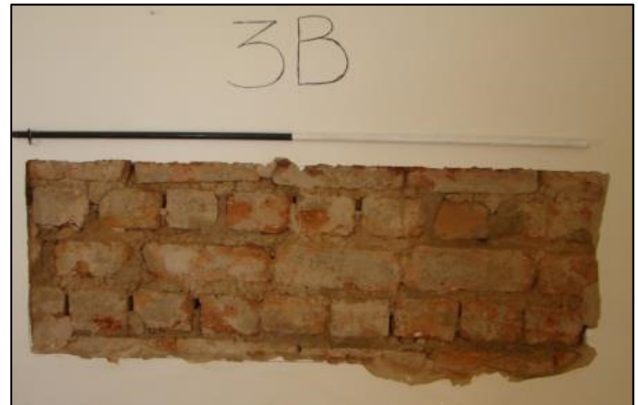
Figure 32: Standard size red brick with grey mortar – English bond.
