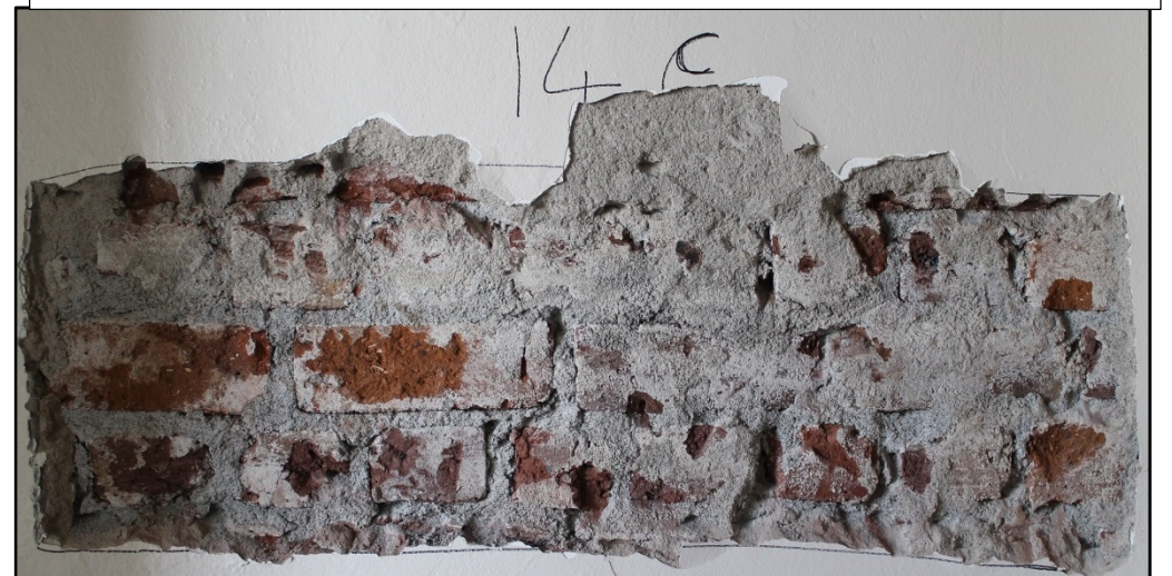
Figure 43: Fired regular red bricks with red mud mortar from plaster strip 14B (same as 14 A). The wall is built in English bond.
