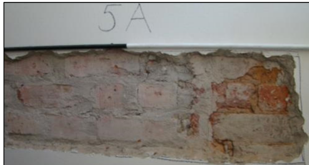
Figure 35: Strip 5A above shows sections of soft red brick and clay mortar to the right while the left consists of a harder red brick and grey cement mortar. Figure 36 below from Strip 5B shows mud brick walls and plaster which is held together with chicken wire.
