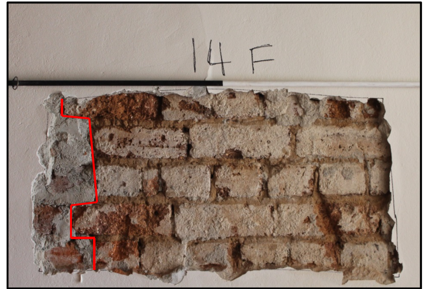
Figures 47: Plaster strips 14G and 14F indicating an aperture in the wall which has been filled with red brick and grey cement mortar. Figure 48 (below) shows the hard red brick and grey cement mortar exposed by plaster strip 14H. Strip 14I reveals a similar wall.
