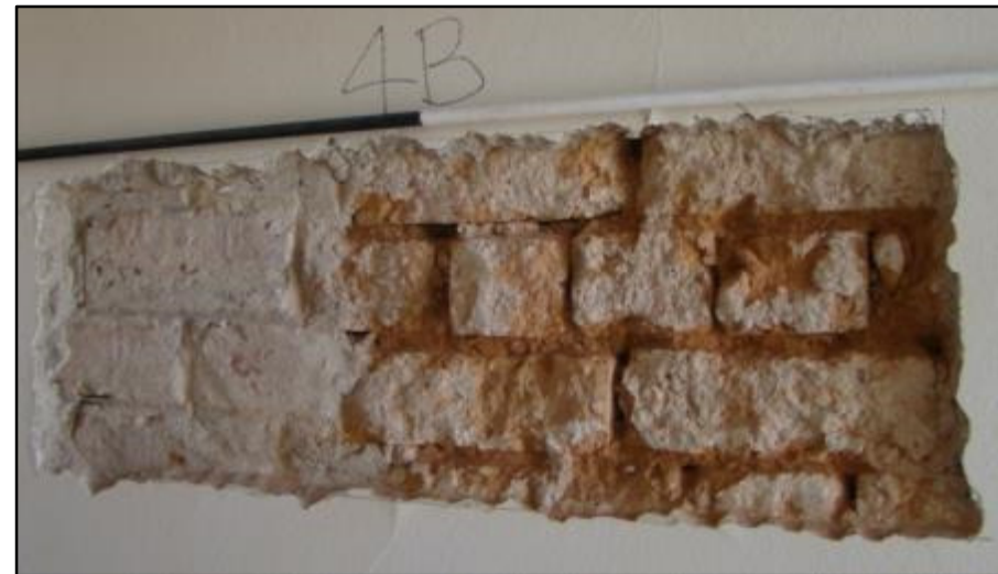
Figure 34: Older red brick and red mortar to the right, recent alteration to left.
