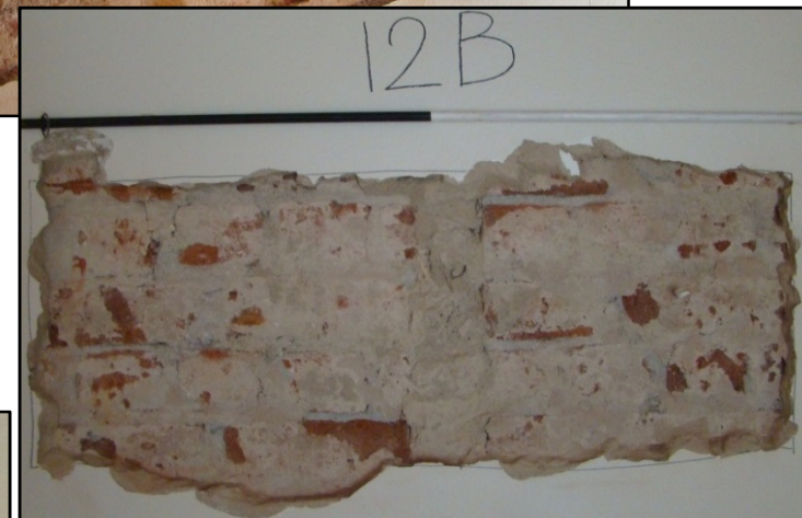
Figures 40: Plaster strips in Cottage 12. All reflect recently constructed walling.
