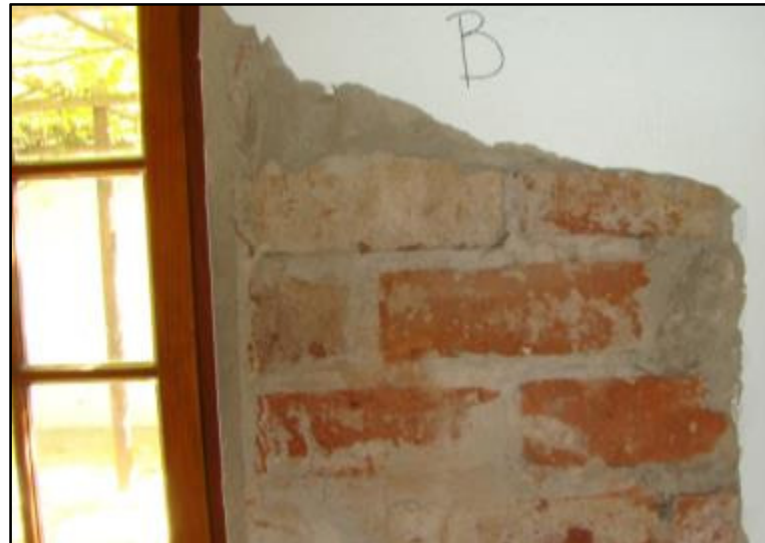
Figure 22: Plaster Strip A between the window and the door on the north facing wall of the southern wing. Note the standard-shaped, fired bricks and grey cement work around the window and door, but the larger and softer red bricks and red clay mortar between them.
