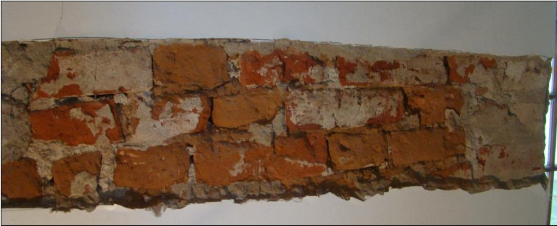
Figure 22: Plaster Strip A between the window and the door on the north facing wall of the southern wing. Note the standard-shaped, fired bricks and grey cement work around the window and door, but the larger and softer red bricks and red clay mortar between them.
