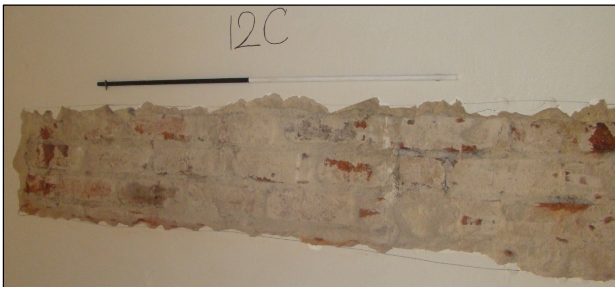
Figures 40: Plaster strips in Cottage 12. All reflect recently constructed walling.
