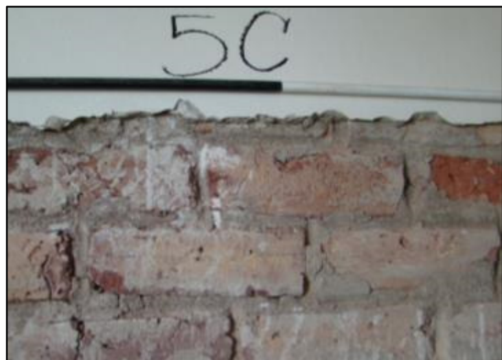
Figure 37: Strip 5C to the left shows a fired red brick wall with grey cement mortar.
