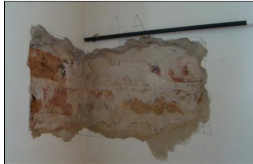
Figure 33: Plaster Strip 4A in corner of room.
