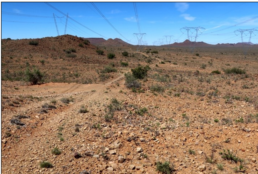
Figure 10: View south-westwards along the main grid connection corridor on Nieuwefontein 89 showing an extensive blanket of rubbly quartzitic surface gravels in this upland area.
