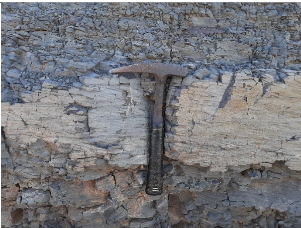
Figure 20 Highly fractured mudstones
