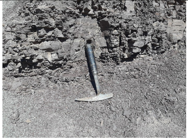
Figure 19 Highly fractured mudstones
