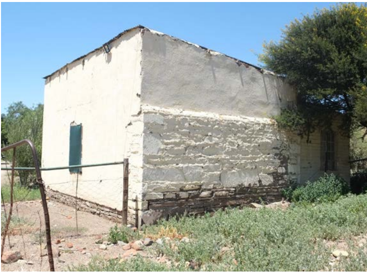
Reverse side of early stone structure
