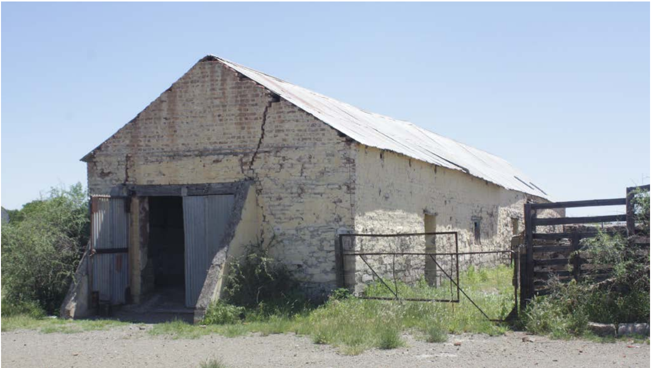
Barn building with fabric layering: stone, brick
