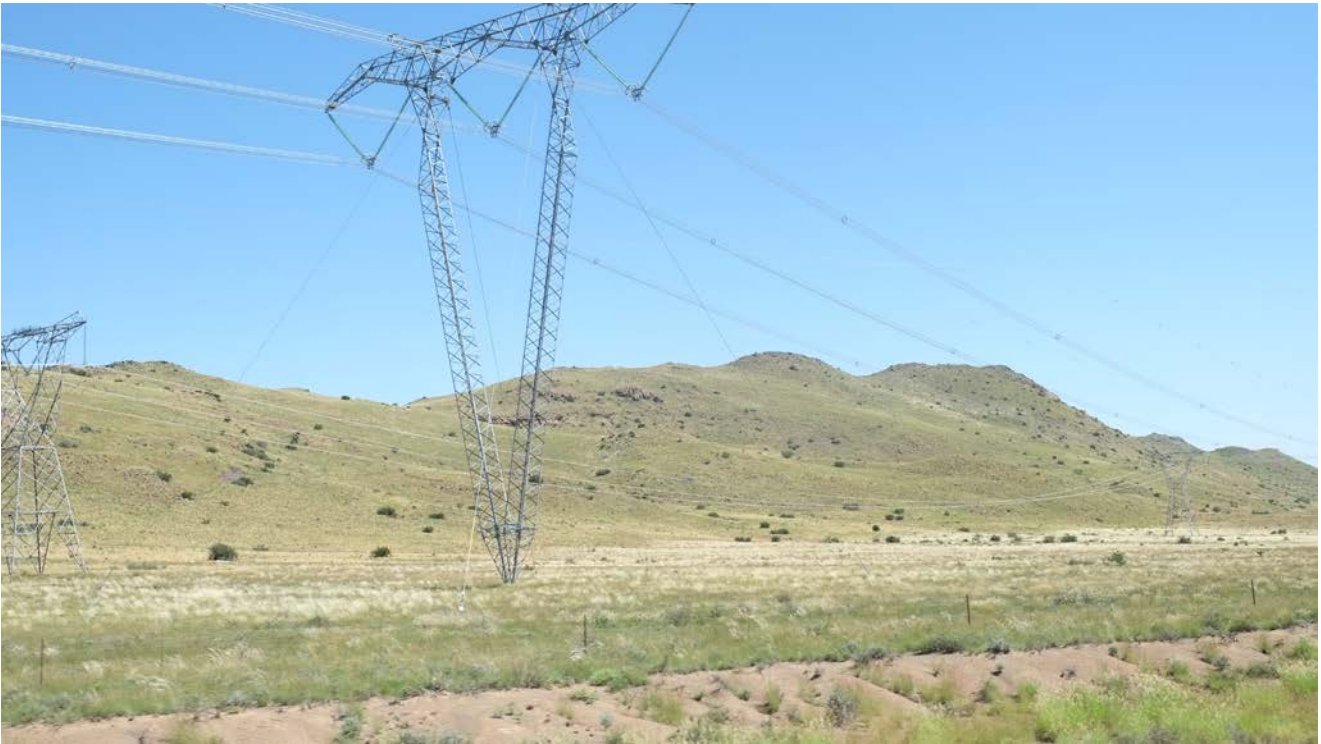
Viewpoint 16: Road south from Nelspoort toward Beaufort west; Eskom infrastructure.
