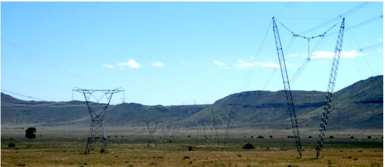
Viewpoint 5: View south, two generations of power pylon extend over ridgeline.
