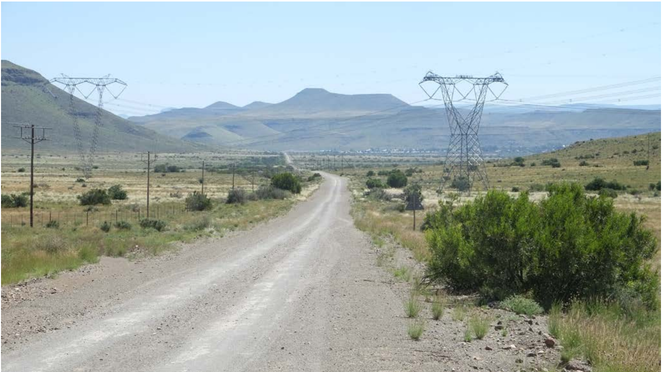
Road south from Nelspoort toward Beaufort west; Eskom infrastructure.
