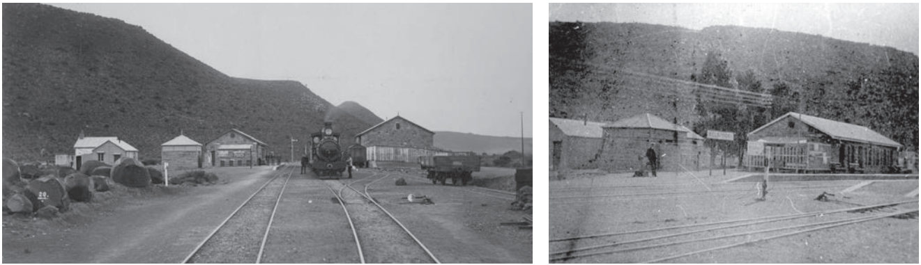
Figure 8. Nelspoort Station in 1895 (left) and early 20thC (right) (Source: DRISA Archive)
