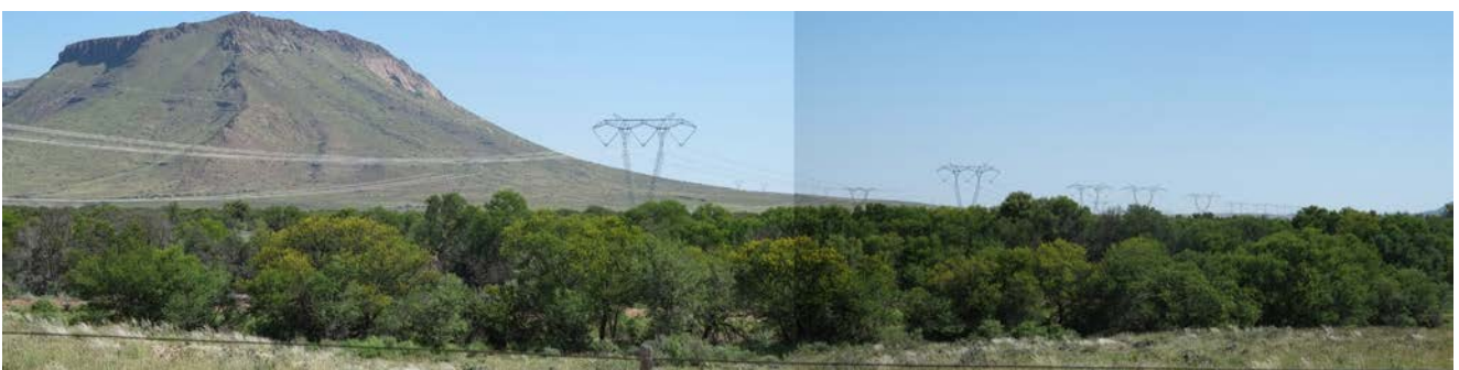
Eskom infrastructure crosses long valley.
