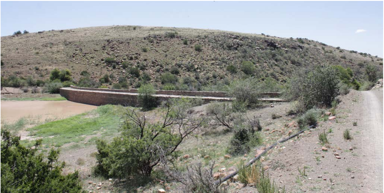
Viewpoint 14: Dam and wall.
