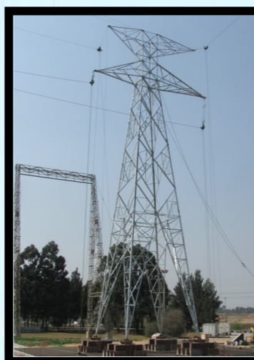
533C HVDC Self Supporting Suspension Voltage: 350 KV Developed: 2006
