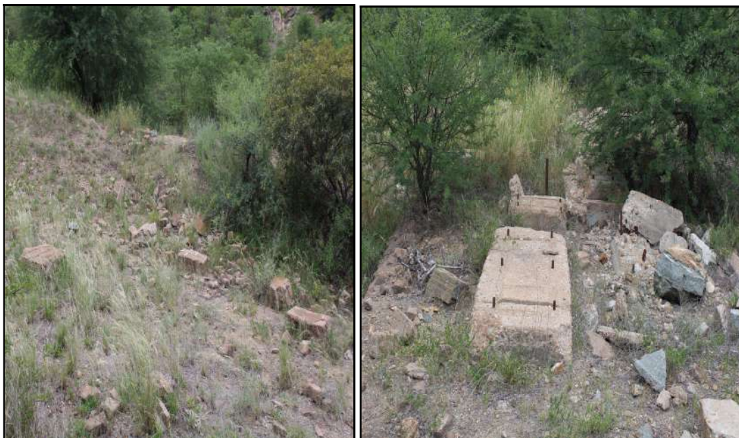
Figure 9: Collapsed mine structures that includes offices and processing plant
