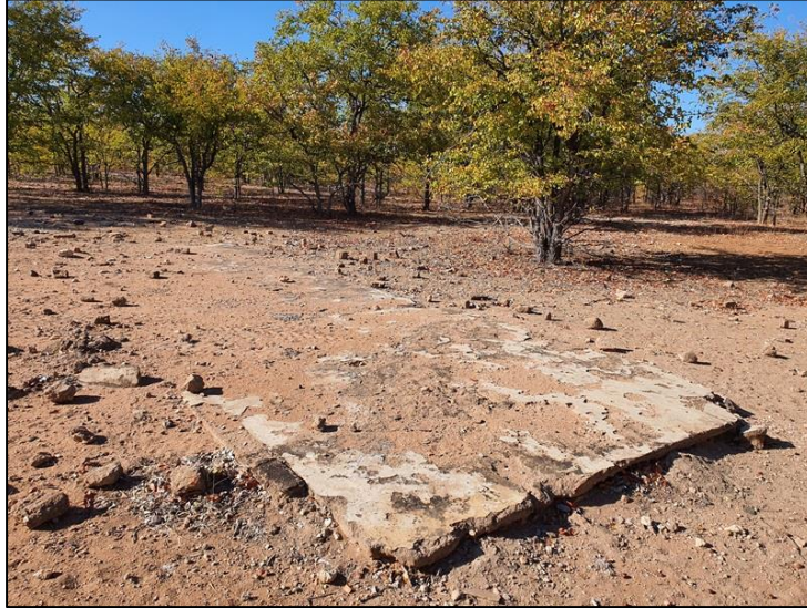
Figure 5-95: View of the poorly preserved building foundation at Site Exigo-BIS-HP01.
