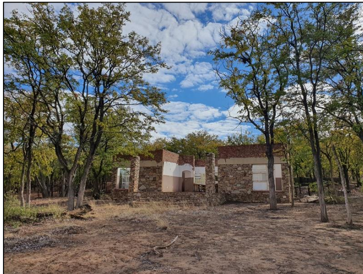
Figure 3-12: View of a dilapidated hunting lodge on Bismarck.
