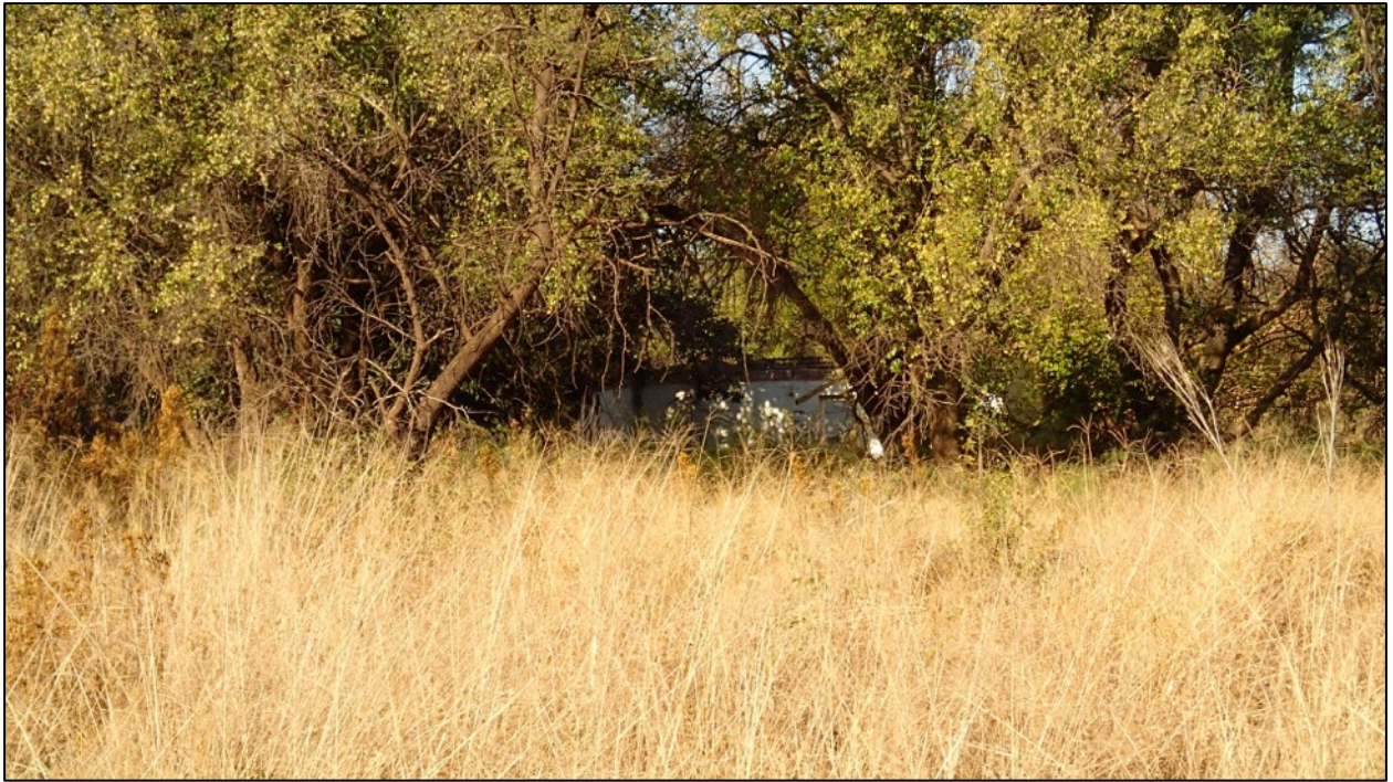
Figure 8: Mud-brick Structure on site
