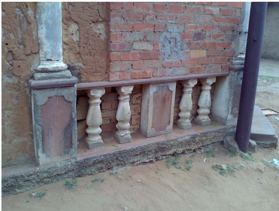
Figure 7: Alterations to the veranda pillars
