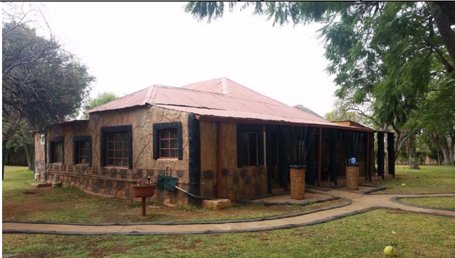
Figure 27: General view of the main farm house (alterations and additions are clearly visible)
