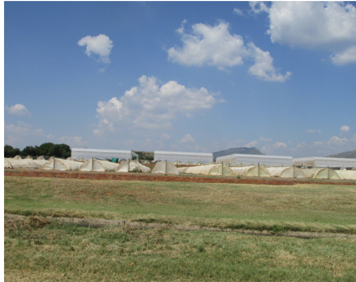
Fig.13: View of some “greenhouses”.
