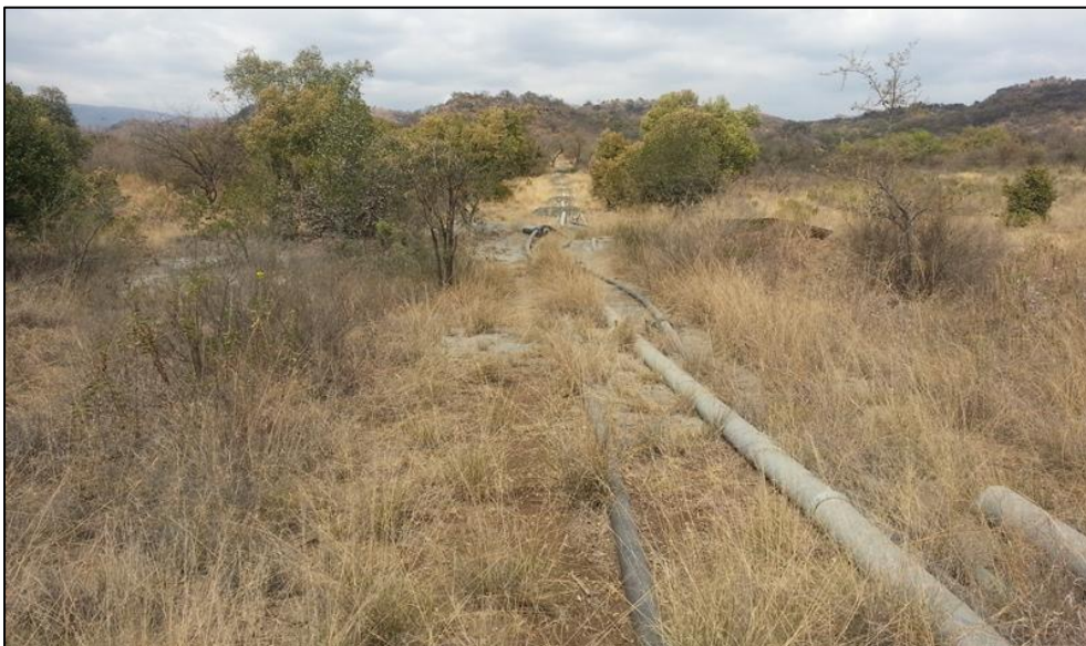
Figure 3-21: Water runoff pipelines along the eastern periphery of the proposed Thorncliffe TSF Site.
