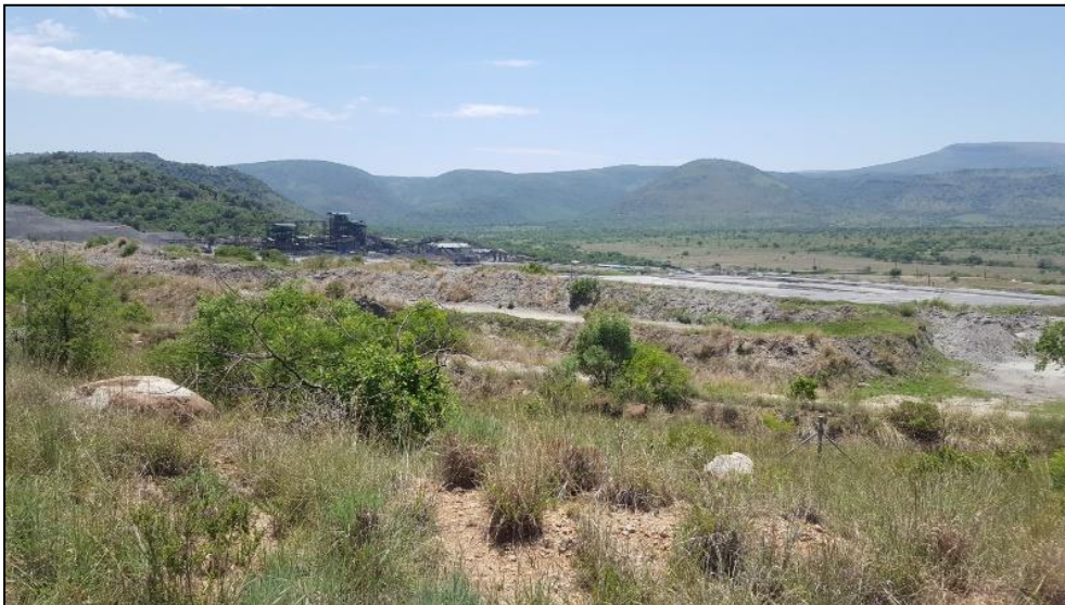
Figure 3-6: View of the current dumps at the site of the proposed Helena WRD.
