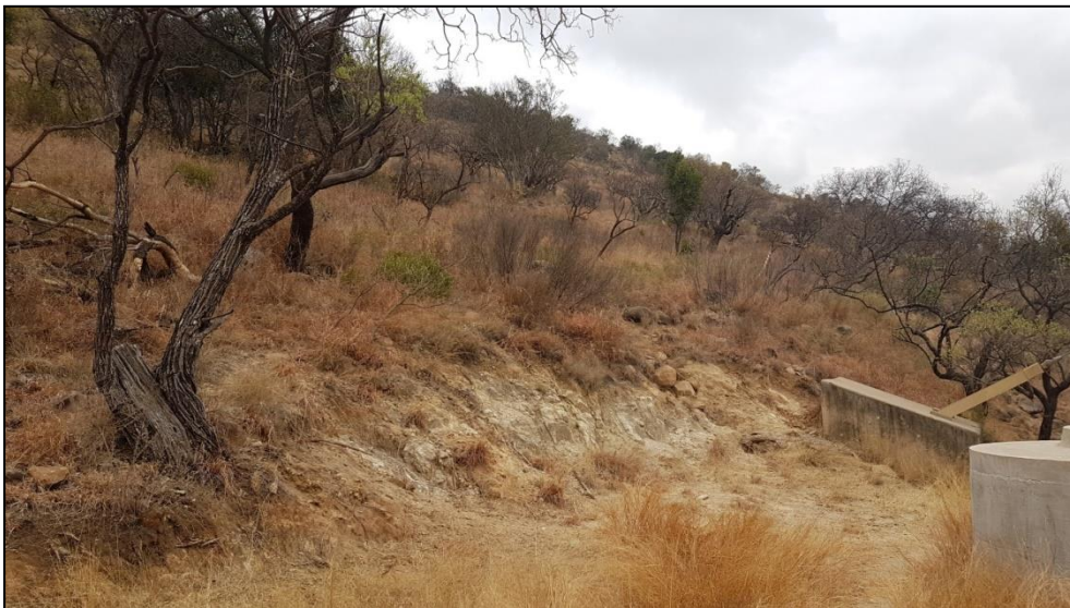
Figure 3-3: View of the Thorncliffe vent shaft location (September 2017).
