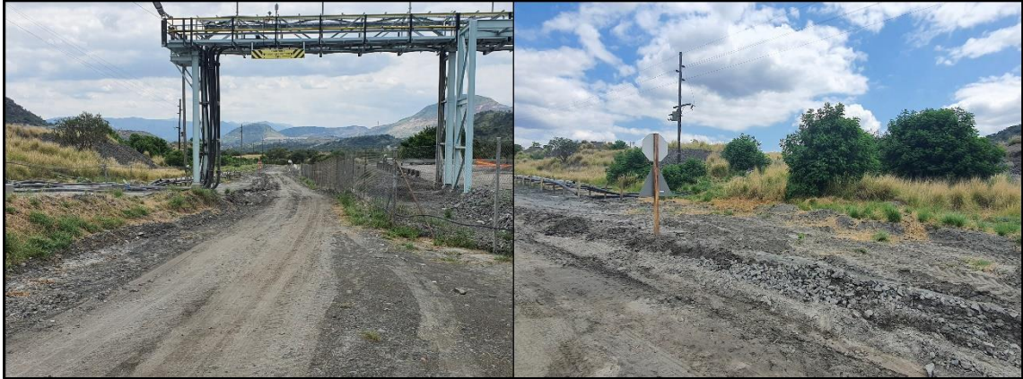
Figure 10: Views of the project area, at the PGM plant extension site Alternative 1 (Preferred).
