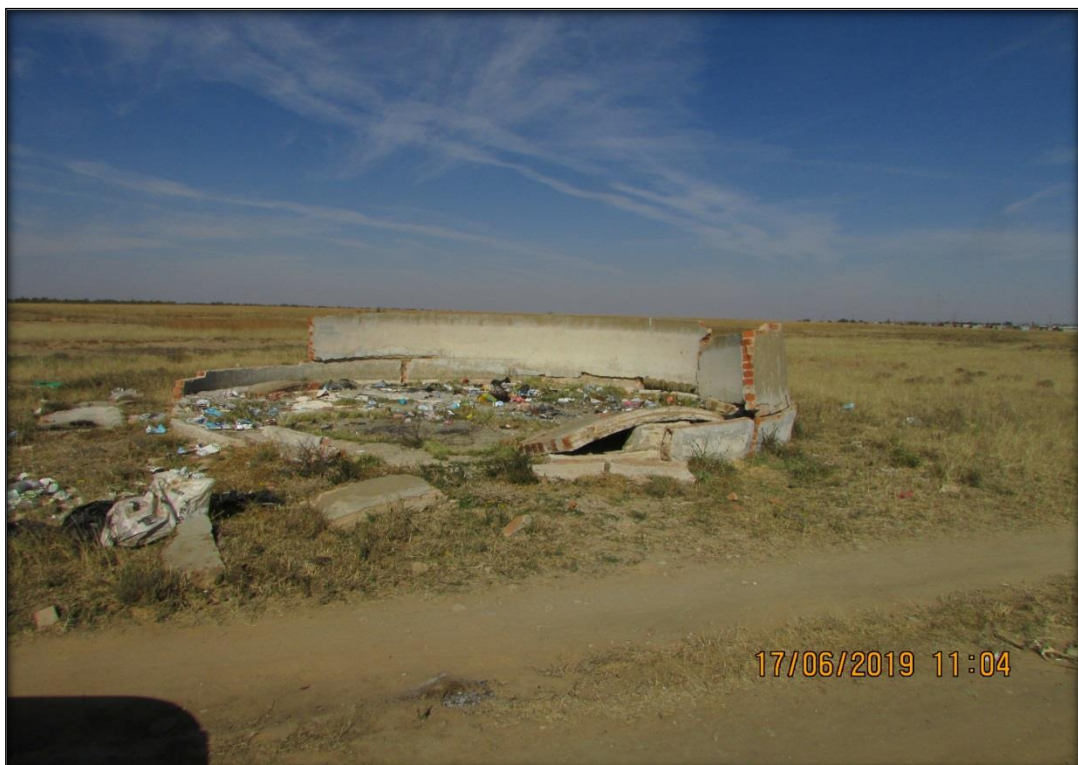
Figure 6: Closer view of the cement farm dam in the area.
