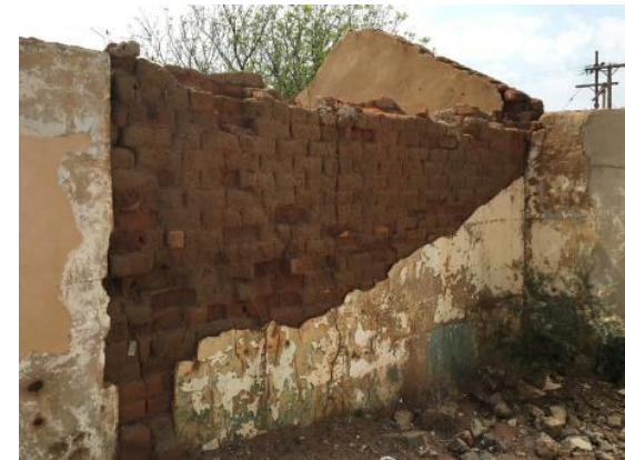
Figure 27: Mud brick internal walls of main house
