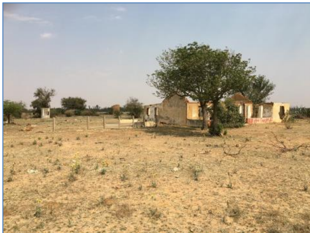
Figure 25: View of farmstead at WB05
