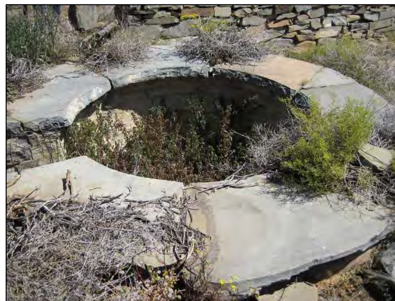
Figure 27 – Stone and cement dipping well
