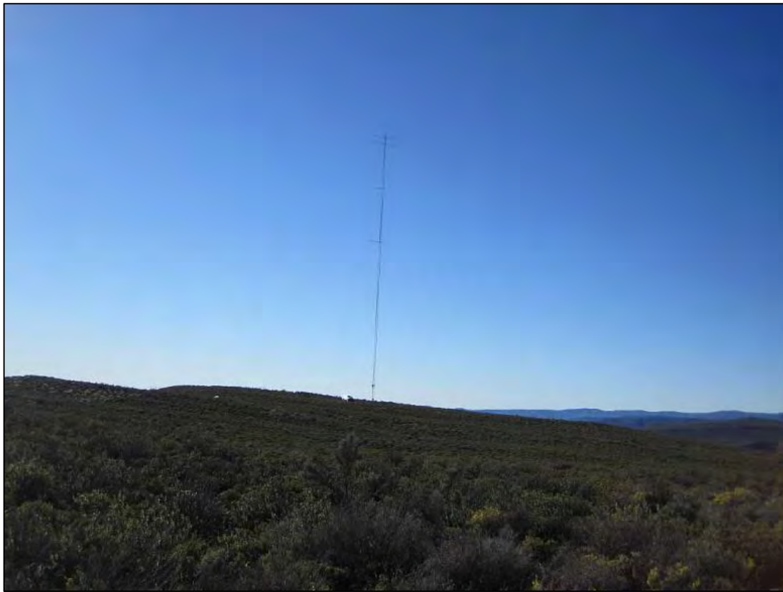
Figure 5 – MET mast on Bloem Fontein RE/192 facing east, S 32° 45' 52,9''; E 20° 16' 54,9''
