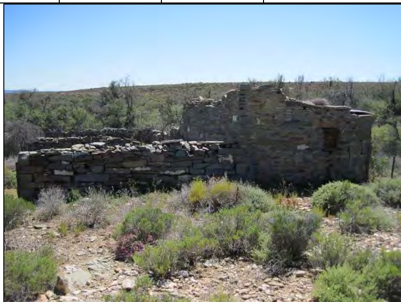
Figure 26 – Small stone house and attached cattle kraal at RKA04
