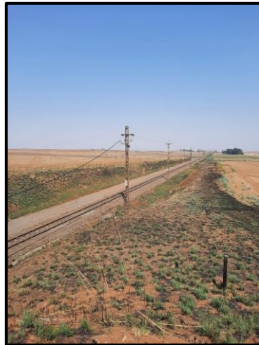
Figure 7.4. Railway infrastructure in the study area.
