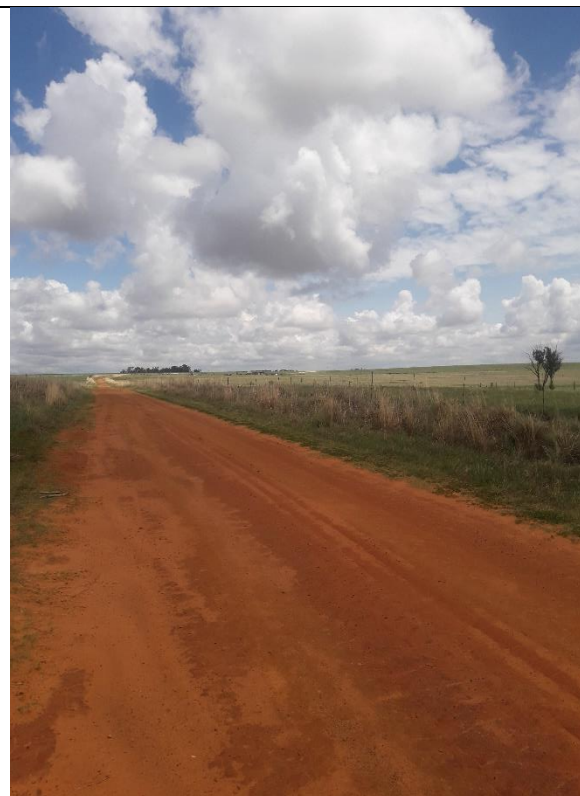
Figure 5B – farm road in southern part of the powerline route. Note generally flat topography and no rocky outcrops
