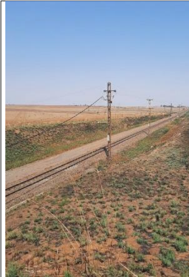
Figure 7A: Railway line close to the southern point where the two routes concur.
