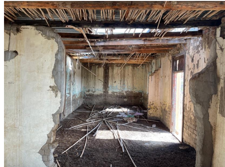
Figure 78: View of the interior of Kh001.
