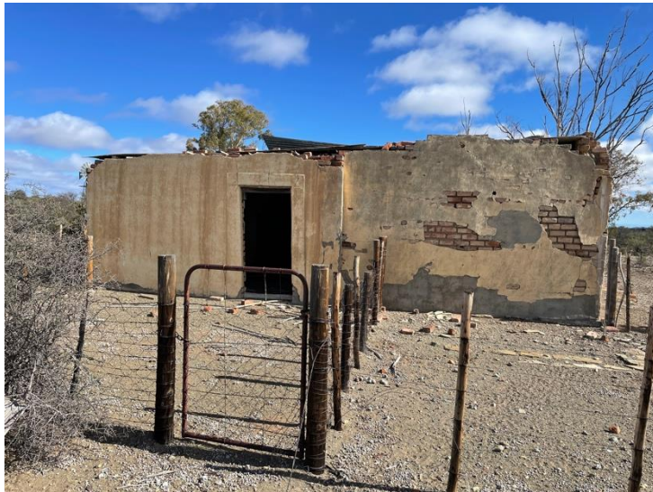
Figure 77: View of Kh001 from the east.
