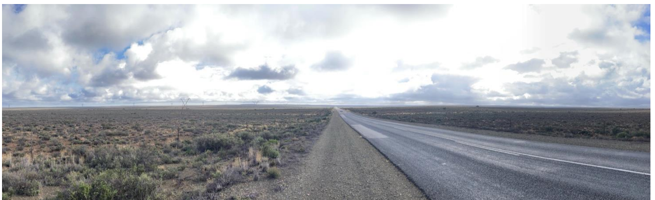
Figure 56: View travelling north on N12 with Koup 1 WEF site on left
