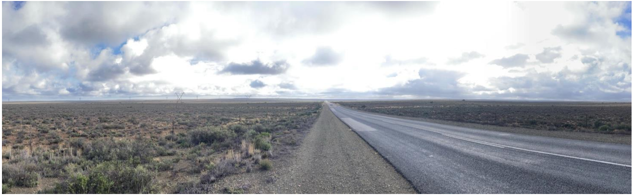
Figure 49: View travelling north on N12 with Koup 2 WEF site on left
