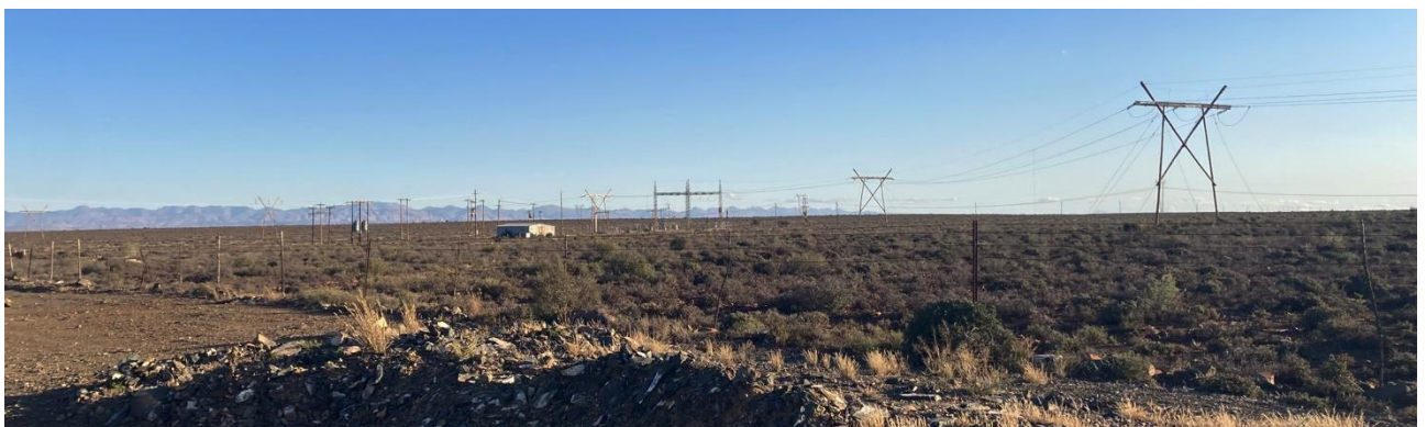
Figure 51: Industrial elements along the N12 south of the Koup landscape.
