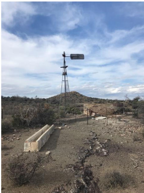
Figure 25: Example of dilapidated windmill and water trough.
