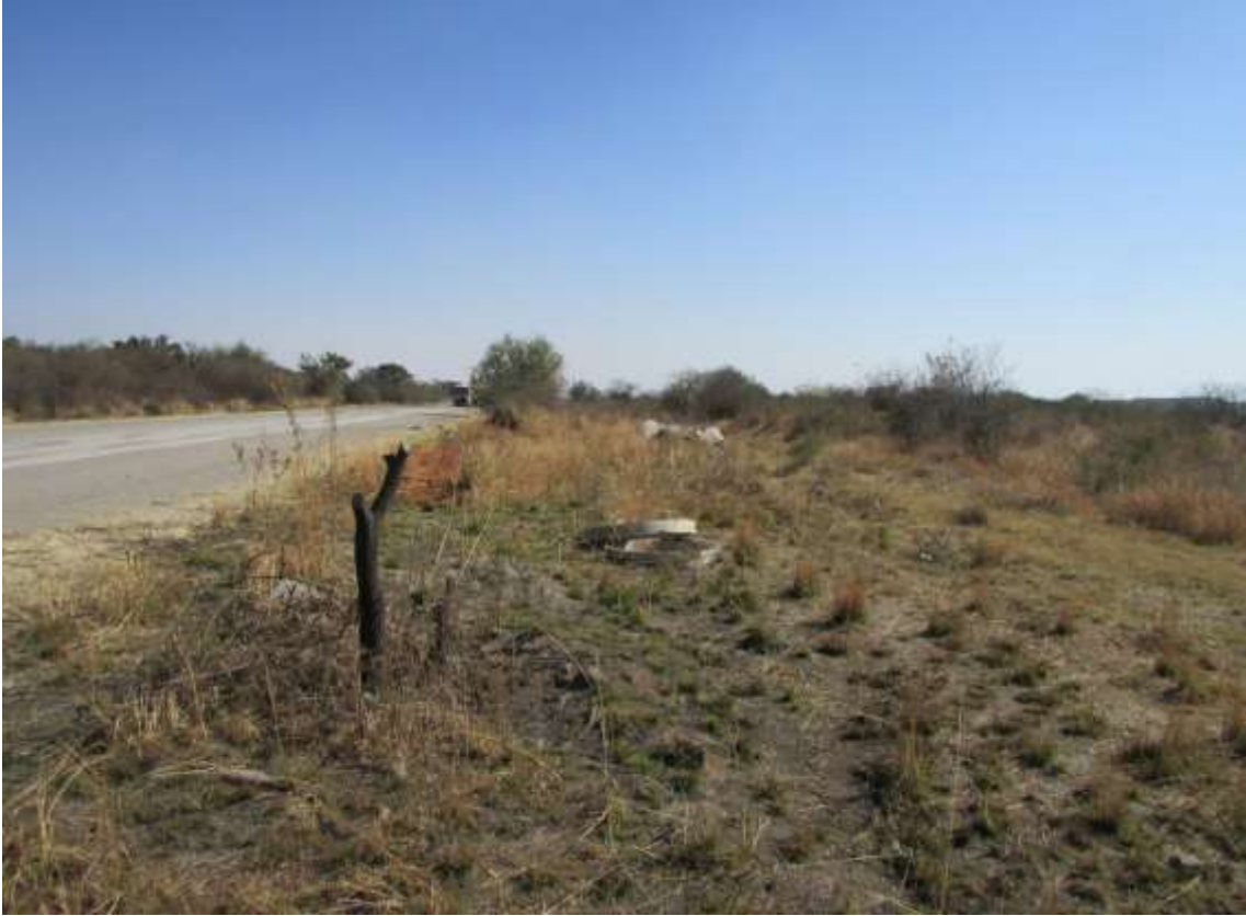
Figure 18: Another view of the Pipeline route with an existing connection visible.
