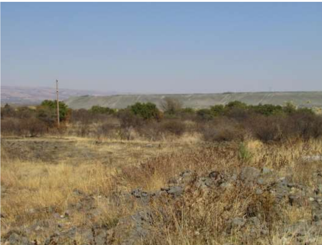
Figure 15: Another view of a section of the new Tailings area with the existing Tailings next to it visible.
