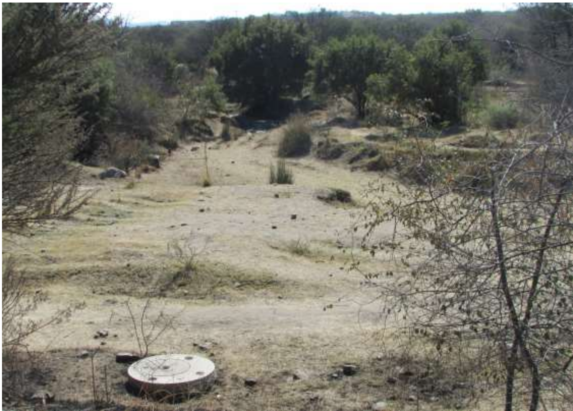
Figure 19: A view of the area of the Pipeline River Crossing. Note the existing connection as well here.
