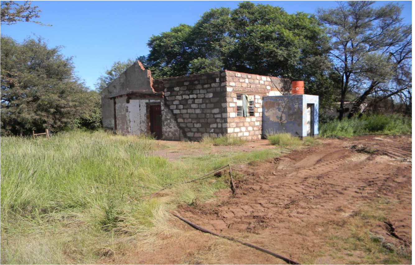
Plate 27: Photo 27: View of the proposed mining right application site (Photograph © by Author 2022)
