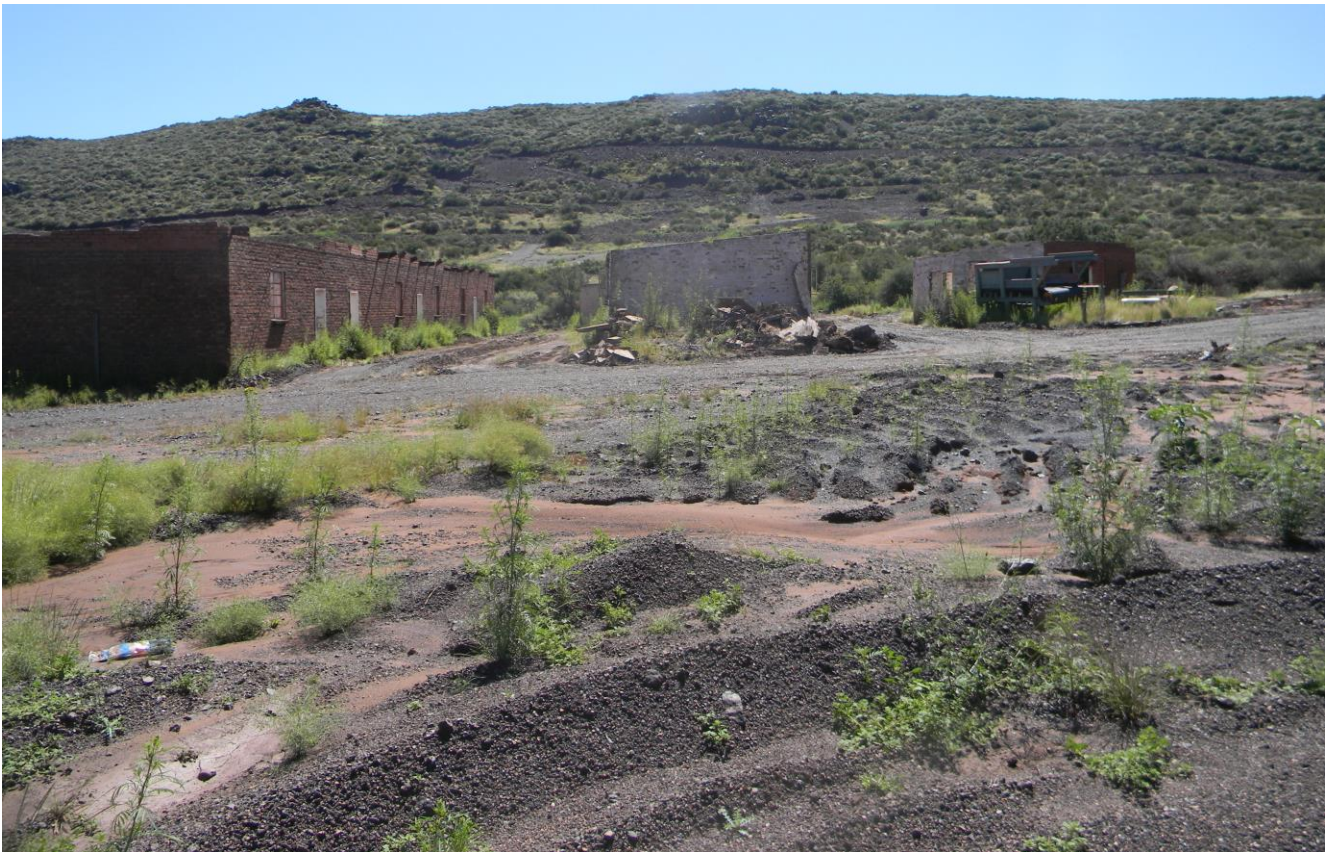
Plate 39: Photo 39: View of the proposed mining right application site (Photograph © by Author 2022)
