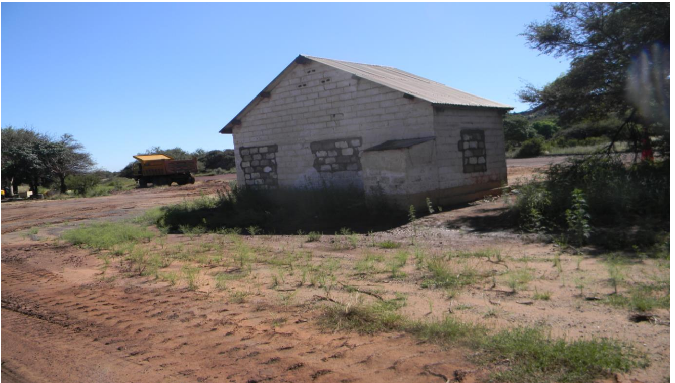
Plate 28: Photo 28: View of the proposed mining right application site (Photograph © by Author 2022)
