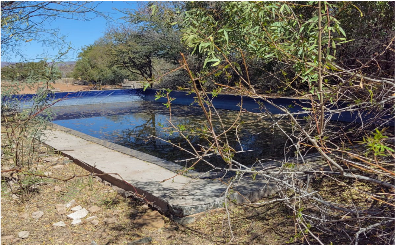
Plate 43: showing water reservoirs.
