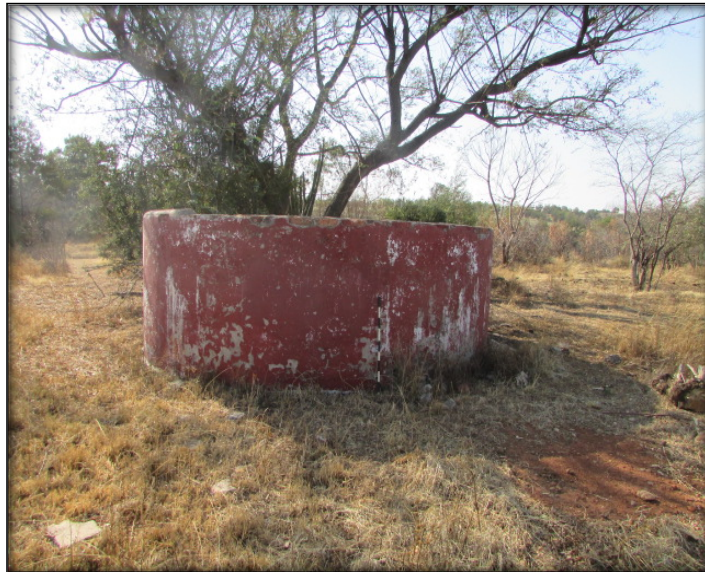
Fig.23: Cement dam on Site 3.
