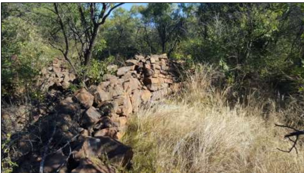
Figure 5-3: Rough stone walling at Site EXIGO-DFM -IA01.
