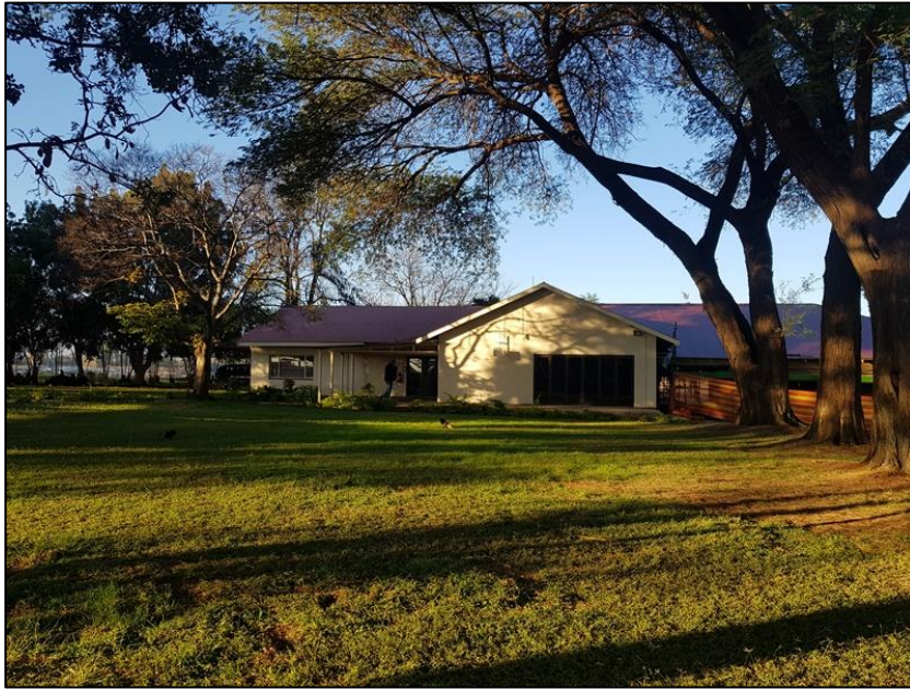
Figure 5-4: A Historical Period building converted into modern offices at the Kroondal Farmstead complex.
